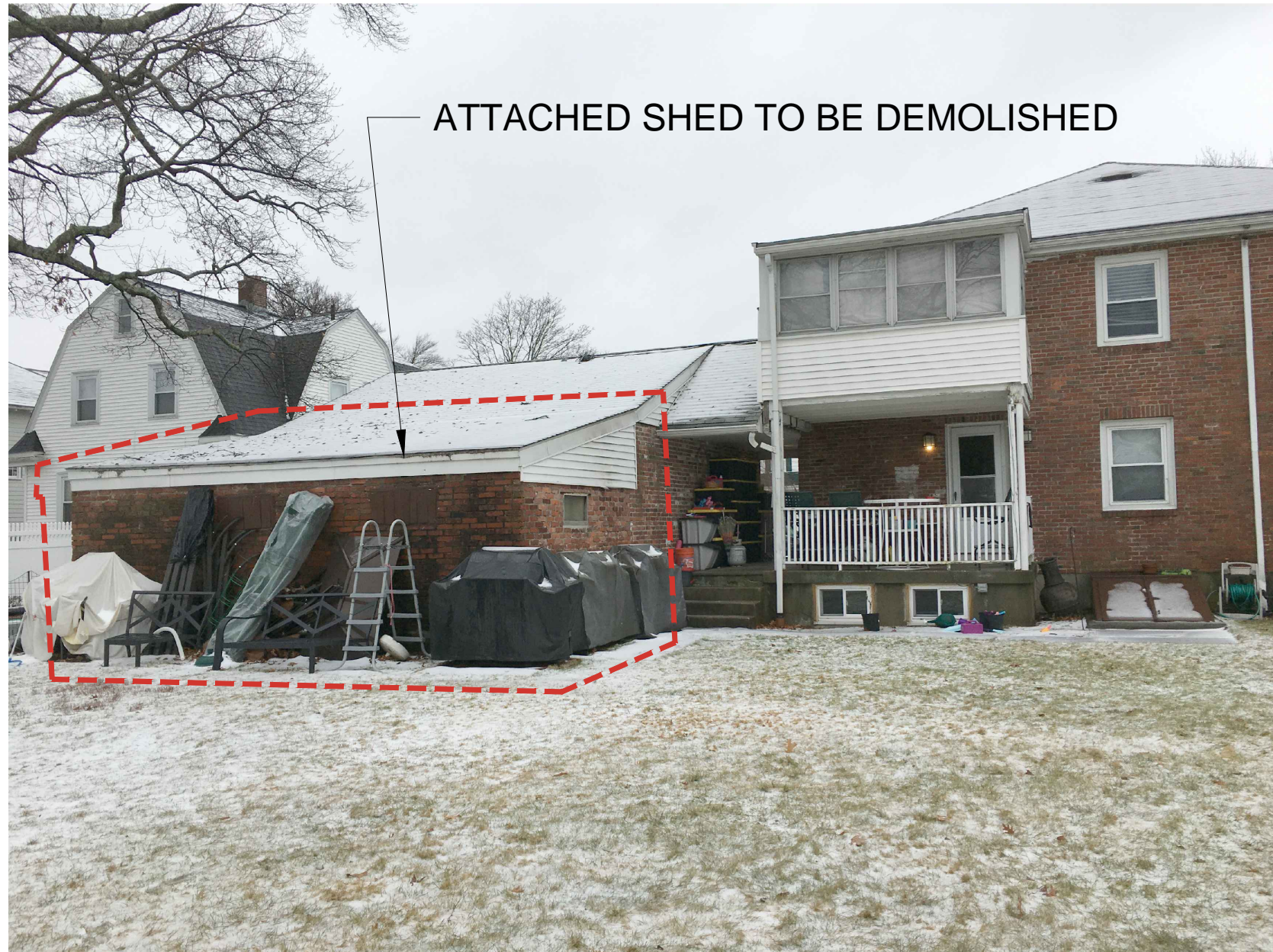
BACK OF HOUSE INCLUDING BACK OF SHED
