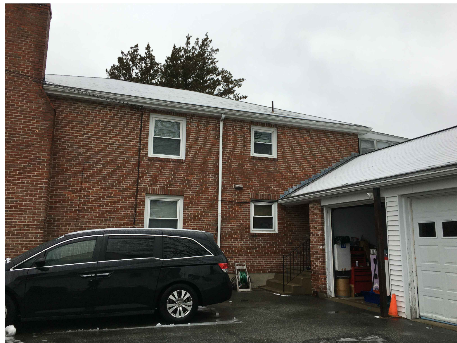
RIGHT FACADE (FROM DRIVEWAY)
