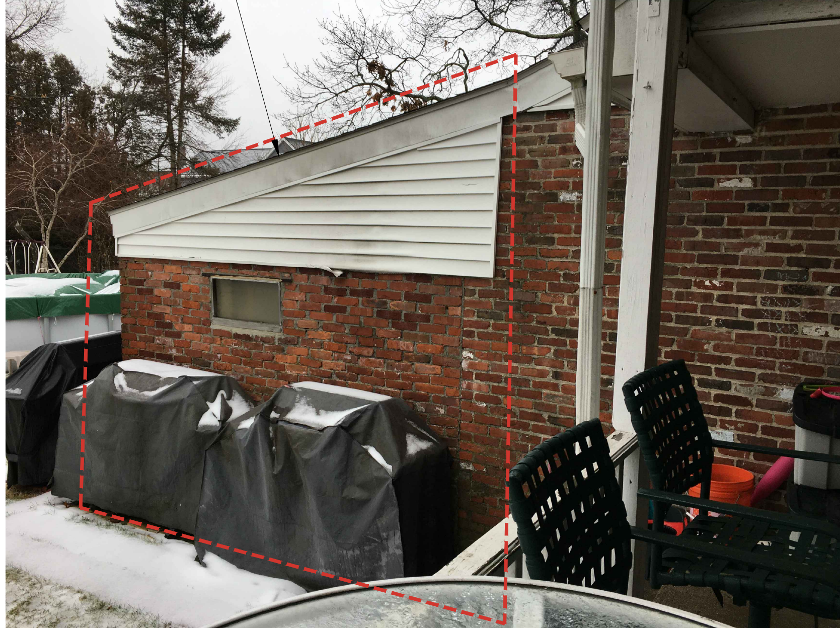
LEFT SIDE OF ATTACHED SHED
