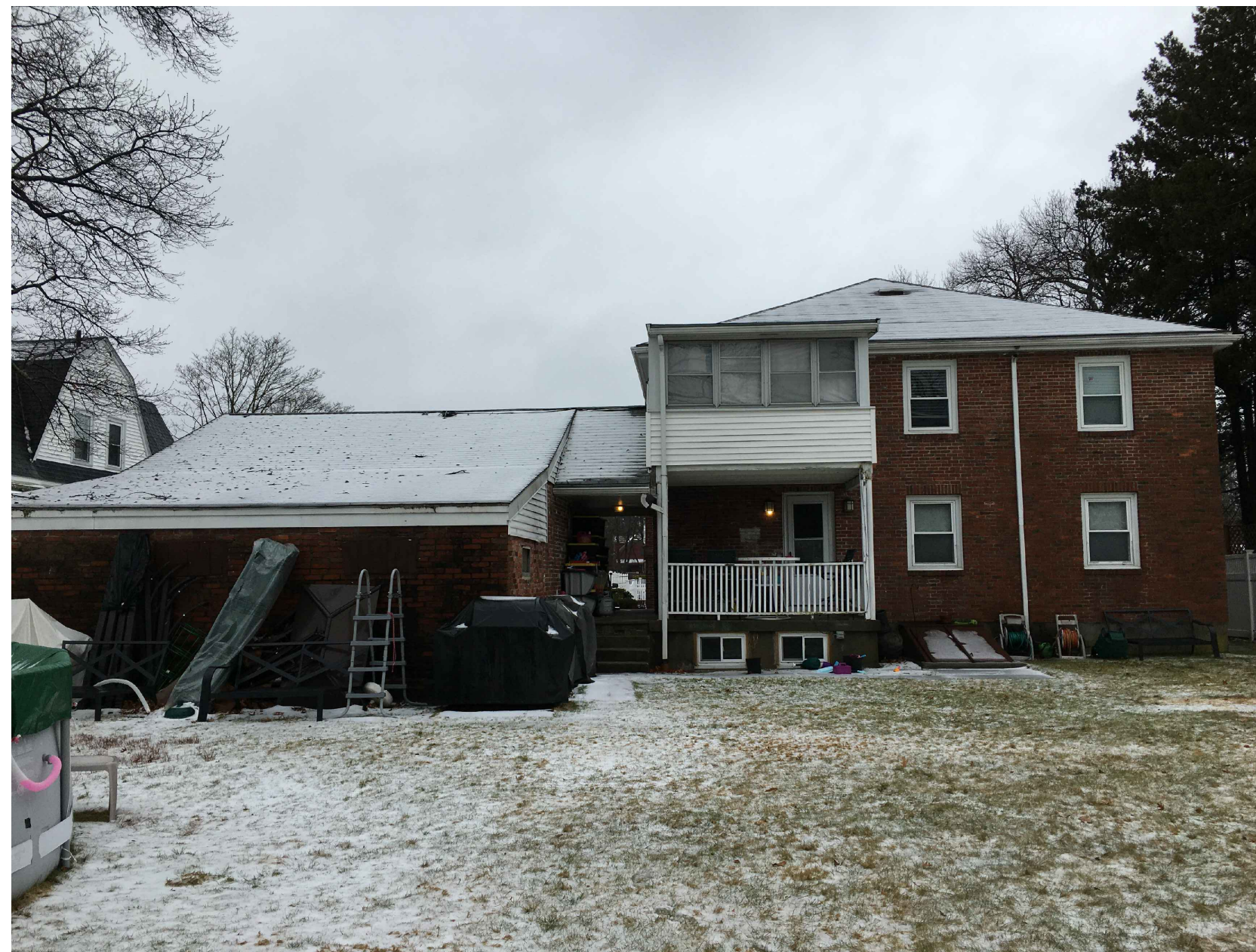
BACK FACADE (FROM YARD)
