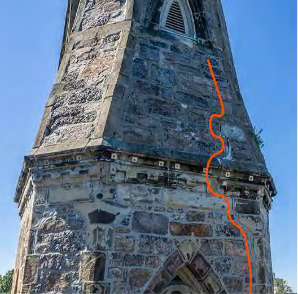
Stabilization – Internal spring-loaded steel reinforcement to resolve structural flaw and resolve issue permanently
