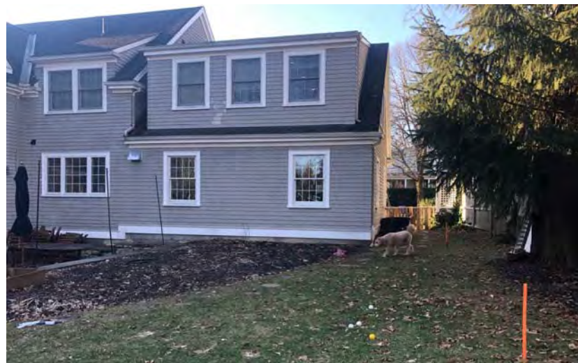
C – Back of Garage from Backyard
