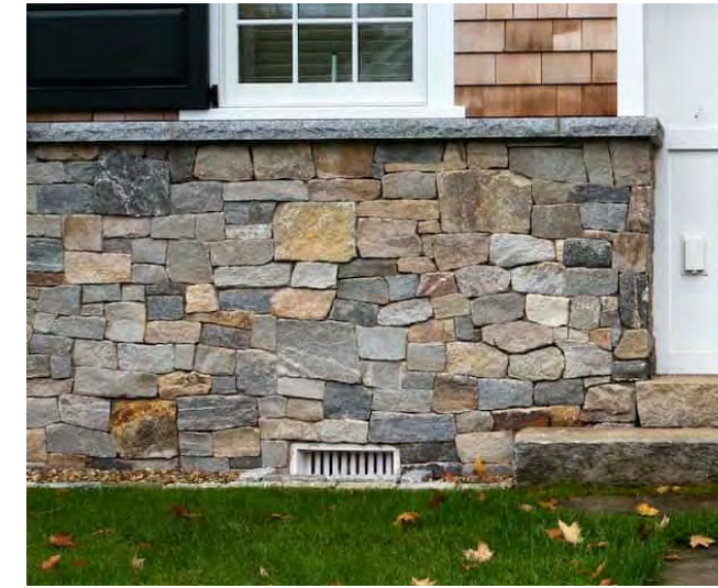
Example of Boston Blend Stone Veneer with Bluestone top Used on retaining wall and riser for two steps down to patio
