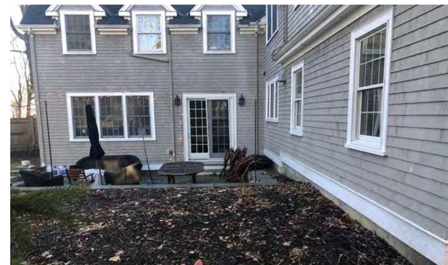
D – Back of House from Side Yard
