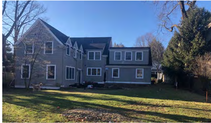
A – Back of House from Backyard
