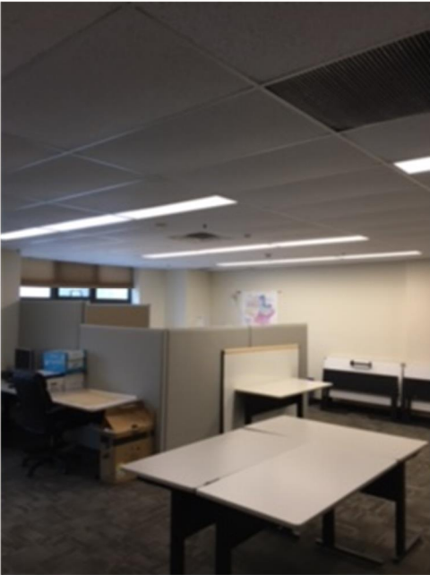
Water Department second floor flat panel LED fixtures
