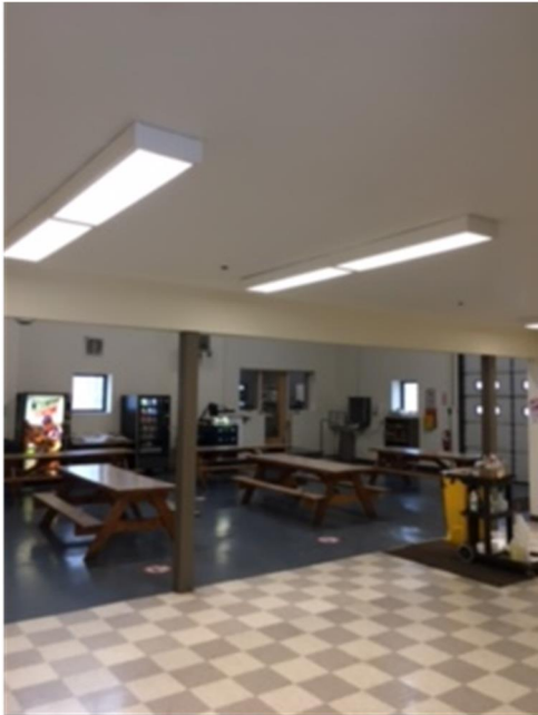
Water Department first floor- replacement LED lamps
