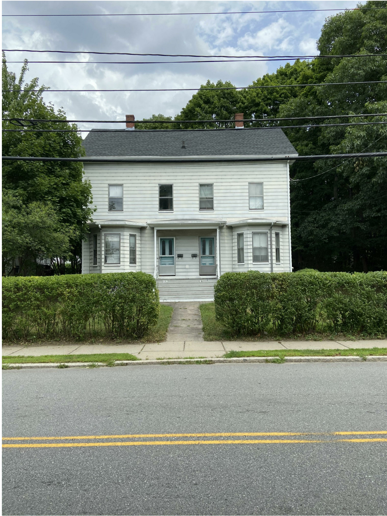
1. EXISTING BUILDING FRONT ELEVATION
