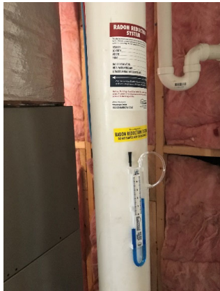
Sealing cracks and gaps and an air purifying unit (APU) (above) Sub-slab depressurization system (SSDS) extraction pipe, pressure gauge, and fan (below)
