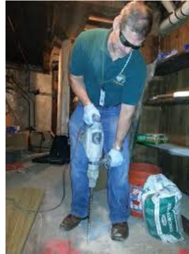
Installation and sampling of a sub-slab soil gas point (above) Canister for sampling indoor air (below)
