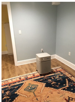
Sealing cracks and gaps and an air purifying unit (APU) (above) Sub-slab depressurization system (SSDS) extraction pipe, pressure gauge, and fan (below)
