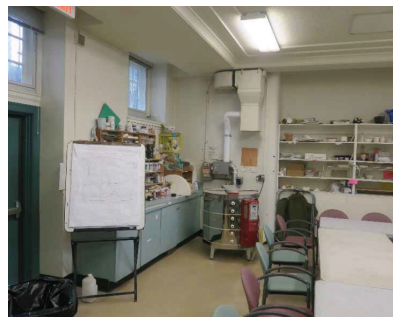
One, or both, of the basement level wings would retain their windows in the proposed concepts that do not cover the front façade of the existing building. This could be secondary use space assuming the elevator is brought to that level.
