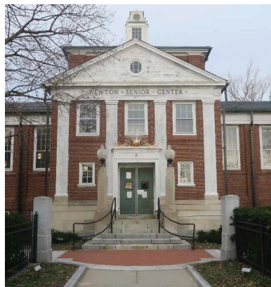
The outside stairs take you up three feet to a landing
