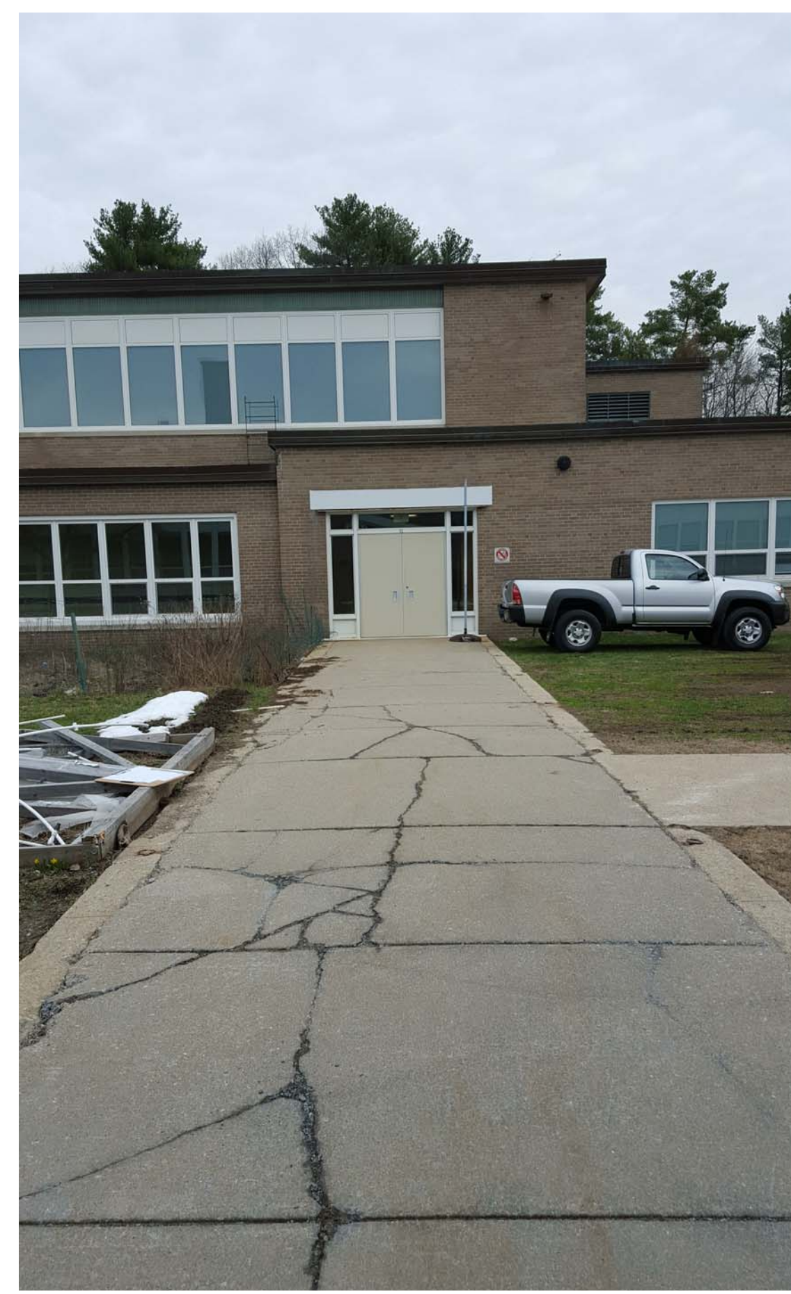
① EXISTING WALKWAY & WEST FACADE
