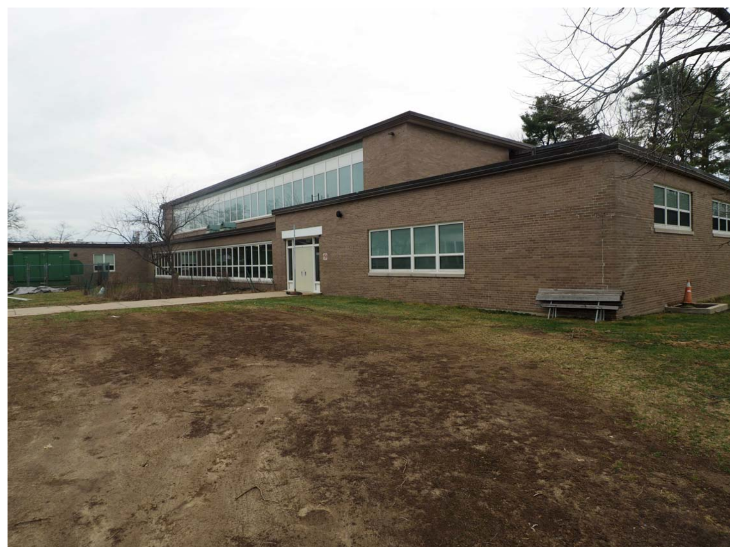
⑤ WEST FACADE - MODULAR SITE IN FOREGROUND
