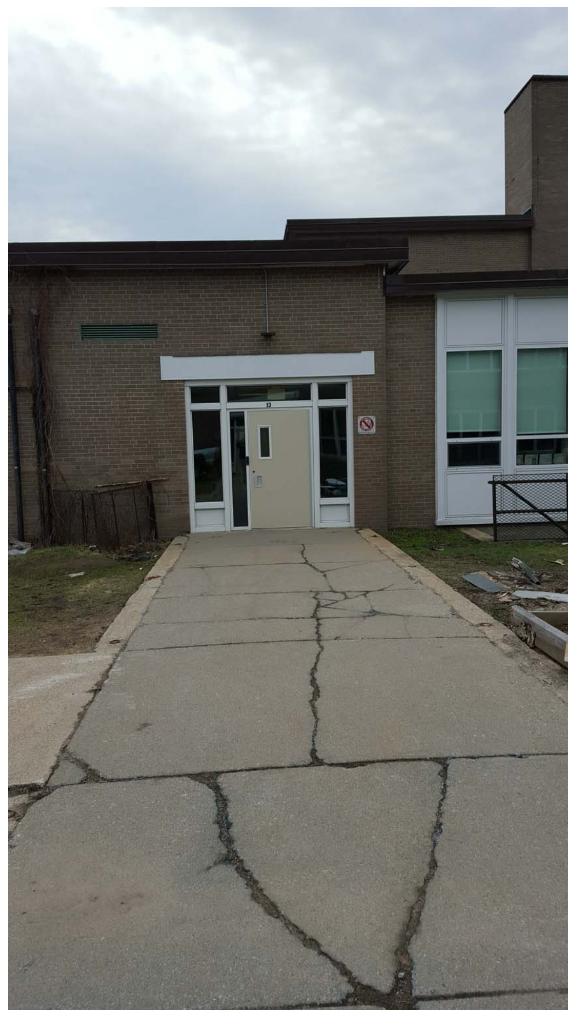
② EXISTING WALKWAY & EAST FACADE
