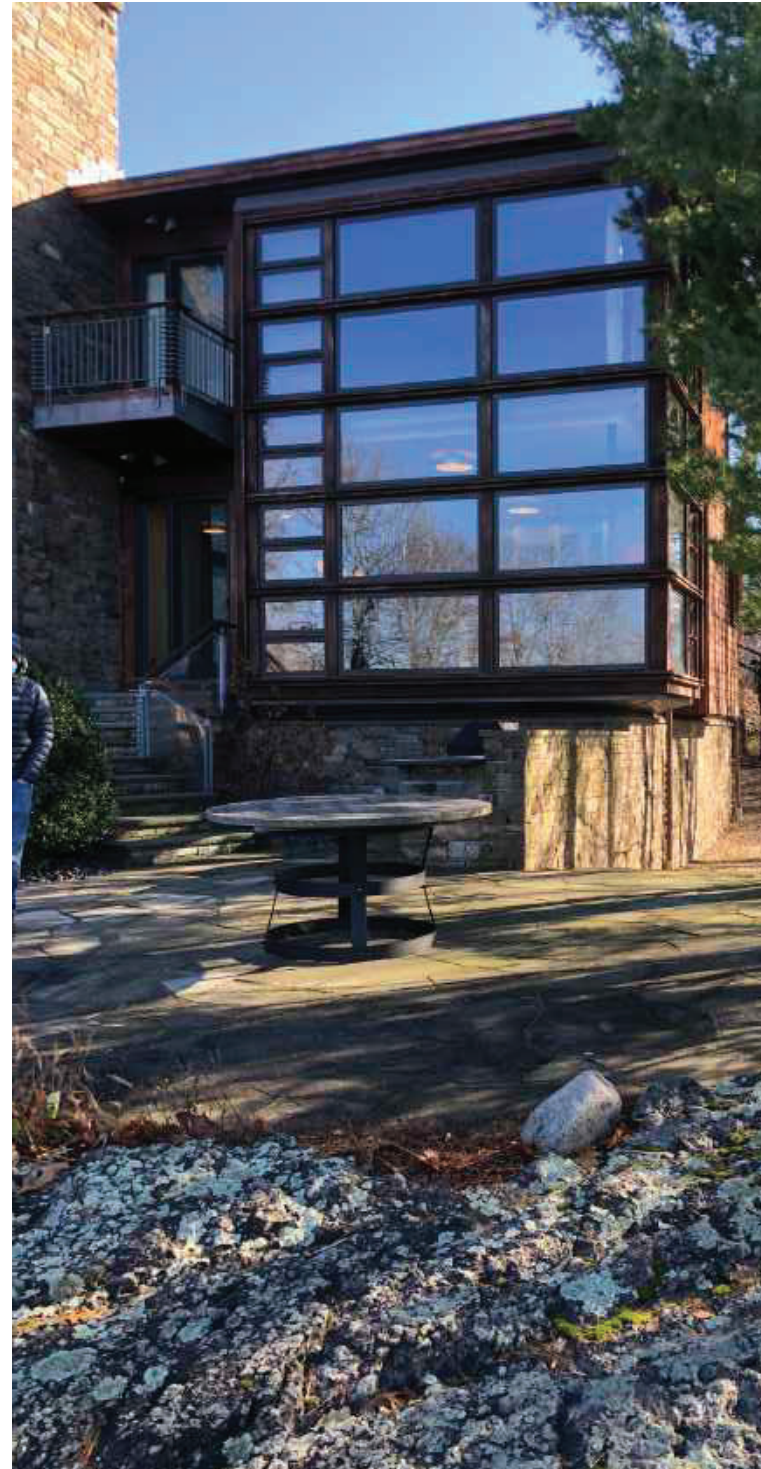
Existing Rear Patio
