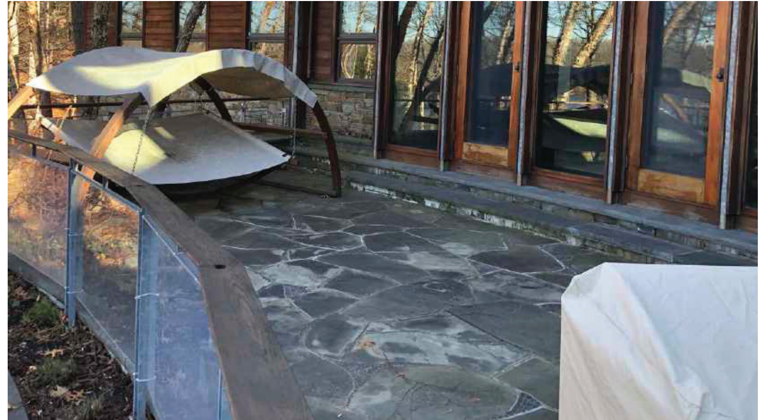
Existing Upper Terrace
