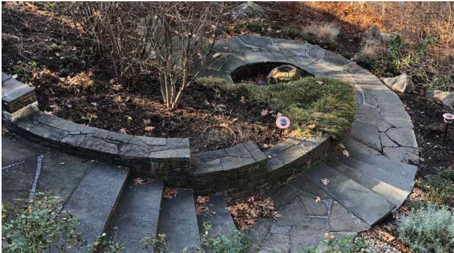
Existing Steps to Lower Patio with Firepit
