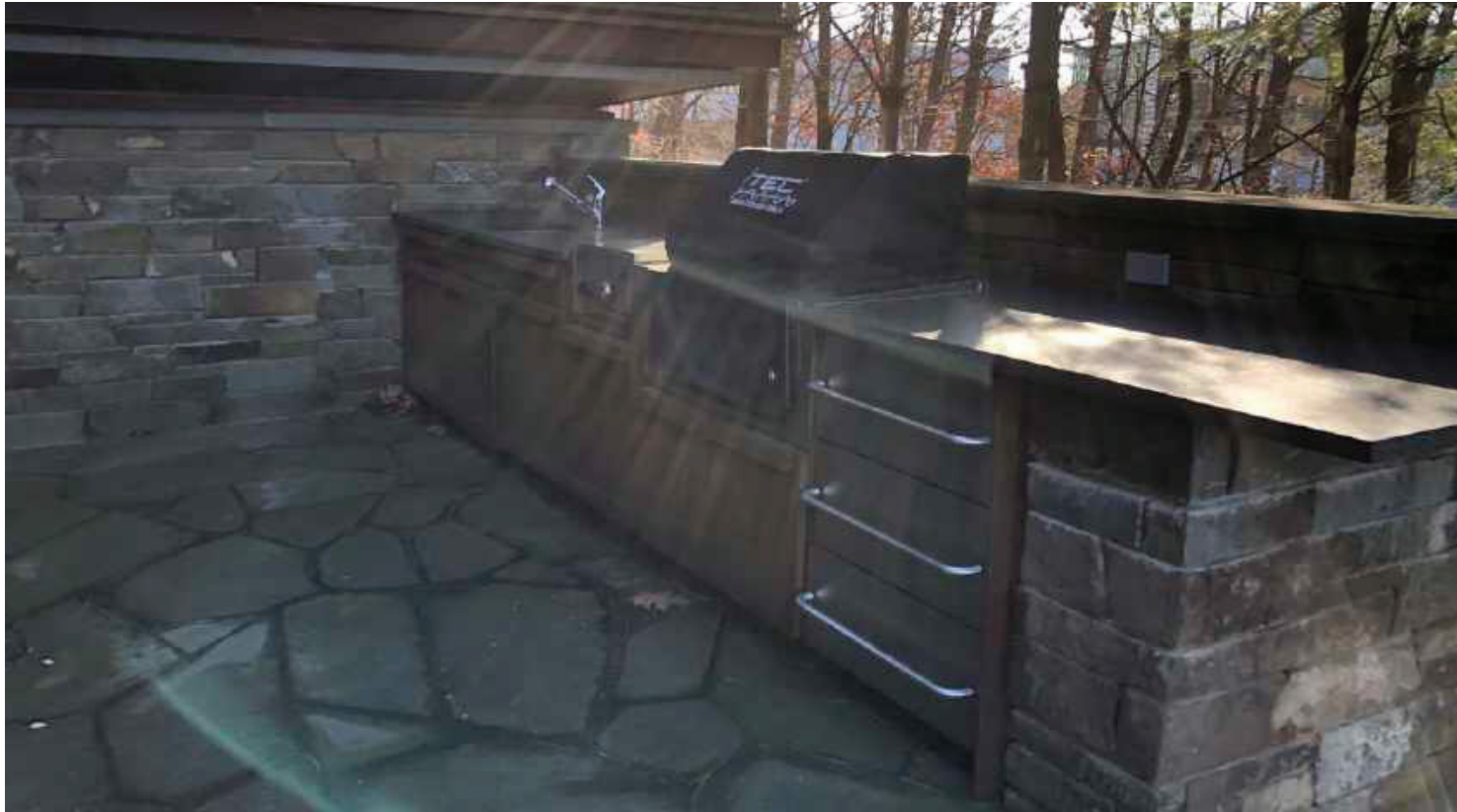
Existing Grill Station
