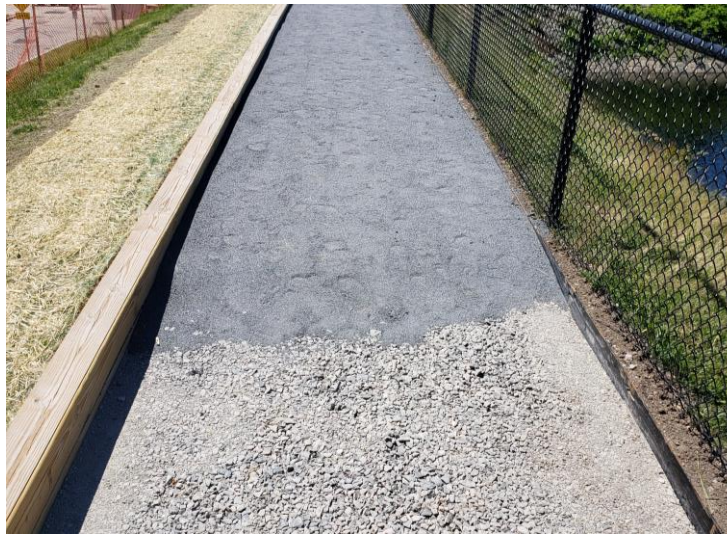
Clockwise from left to right: Timber edge and steel brackets; New stair cheek wall form work and poured concrete; Newly poured and curing concrete stairs; Stabilized stone dust, aggregate base, timber curb and erosion control matting; new granite curbing at accessible parking space
