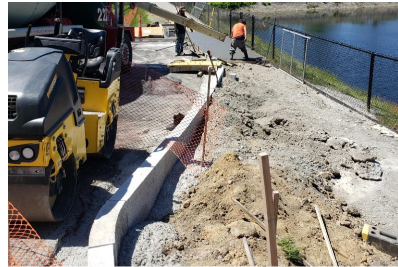
Clockwise from left to right: Timber edge and steel brackets; New stair cheek wall form work and poured concrete; Newly poured and curing concrete stairs; Stabilized stone dust, aggregate base, timber curb and erosion control matting; new granite curbing at accessible parking space
