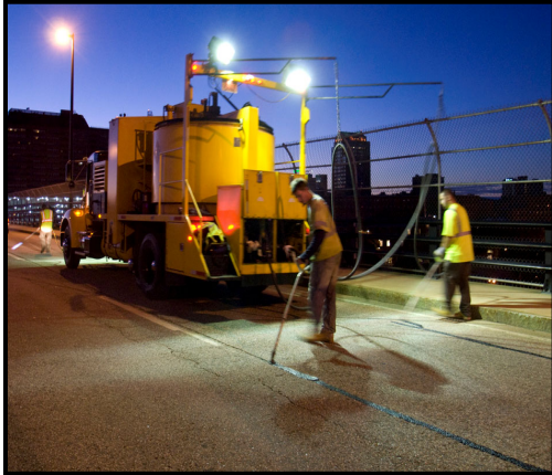
Crack Seal
