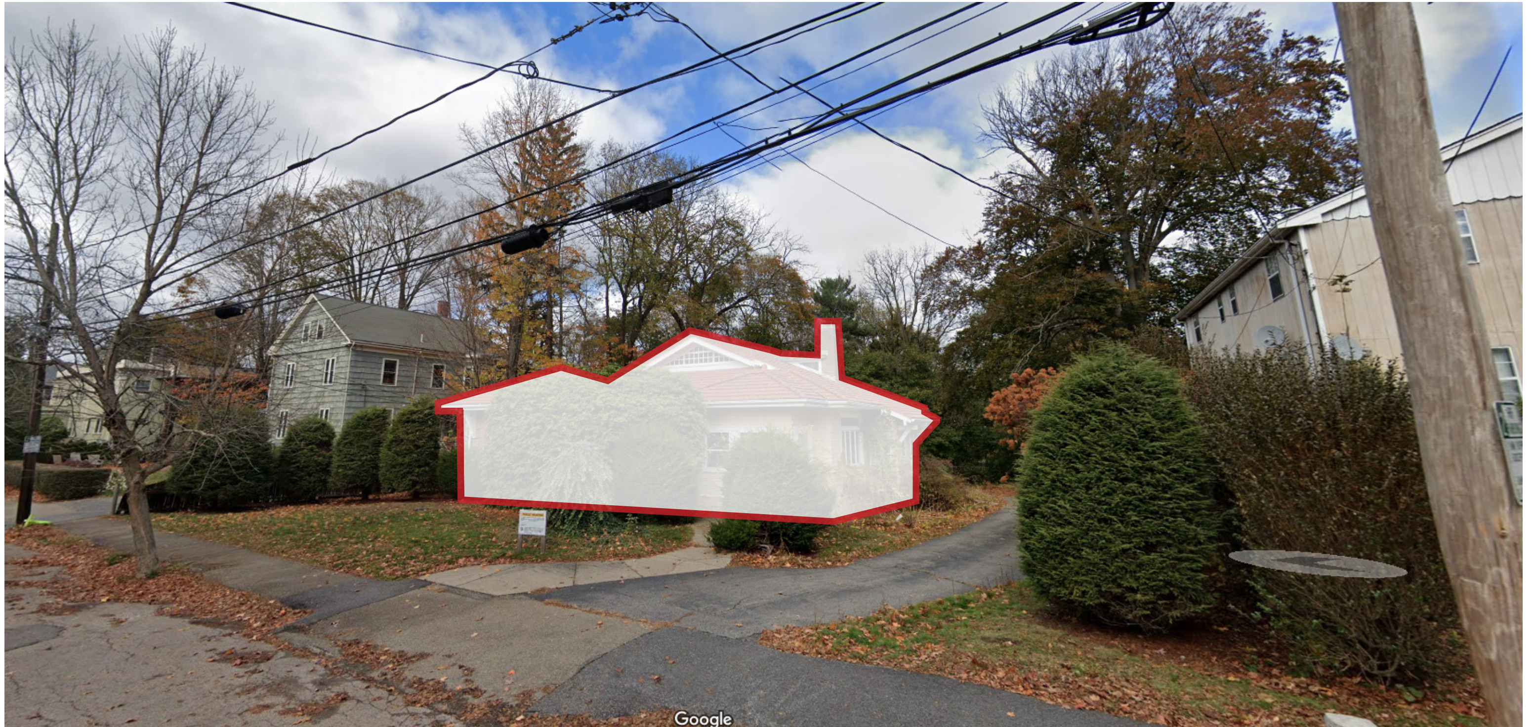
Historic "Aloha" House
