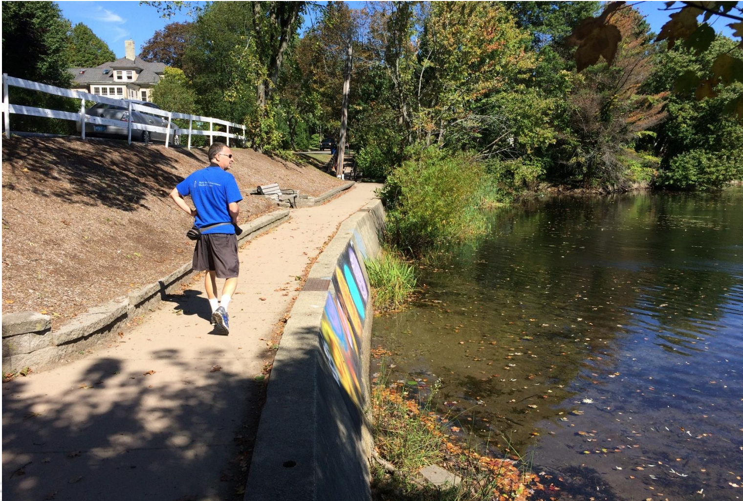
Improvements at the “Fishing Wall”
