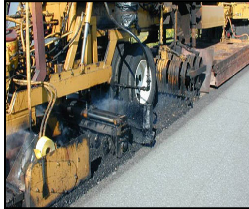
Hot In-Place Recycling
