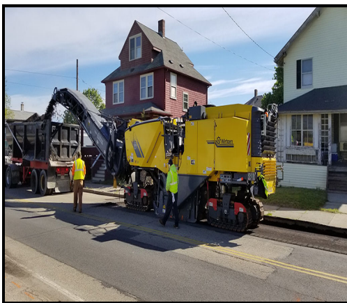
Mill and Overlay
