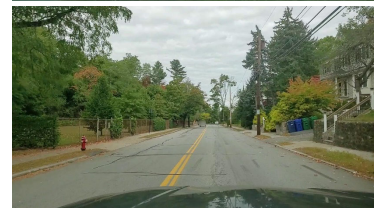
Lowell Avenue Preventative Maint.
