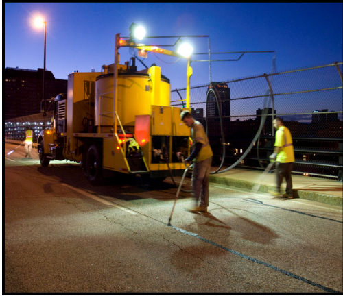
Crack Seal
