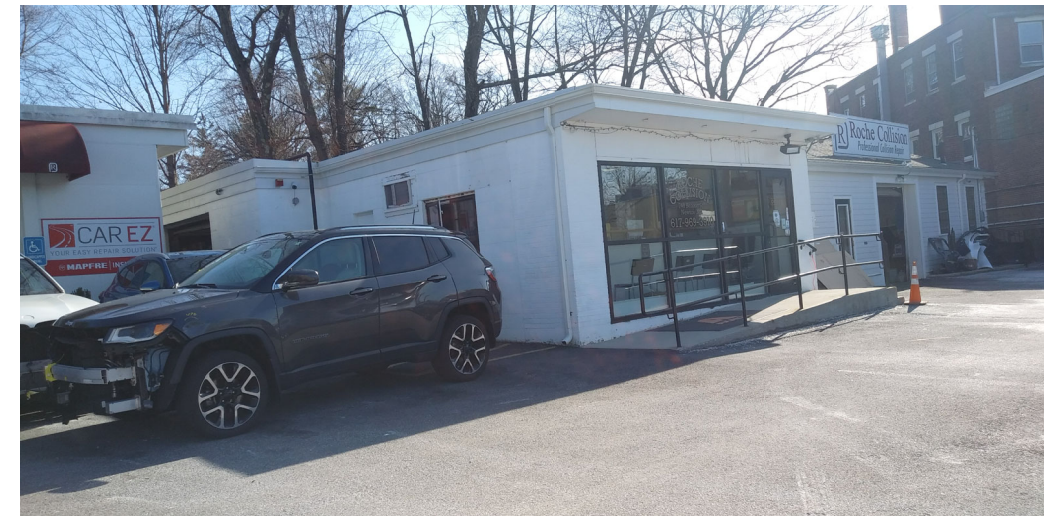
IEWS OF EXISTING BUILDING SCALE : NO SCALE
