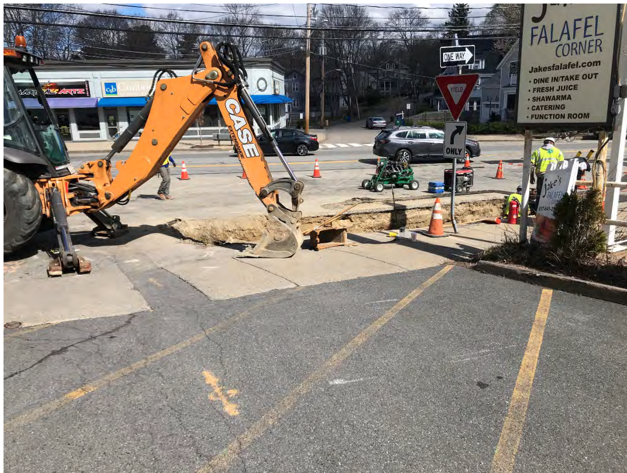
Access Driveway Apron
