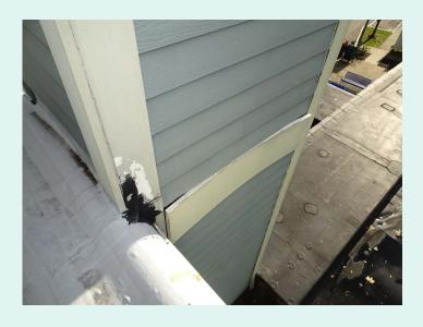
Existing siding and trim has extensive damage and must be replaced.
