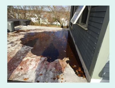
Existing roofs must be replaced. The existing air conditioning system must be removed and all 35 units replaced. The new roof insulation will be increased to R-50, and the new roof will be a white TPO. The existing air conditioning system will be replaced with more efficient condensers. This includes 35 condensers, one for each apartment, and 3 roof top units that cool the common areas.
