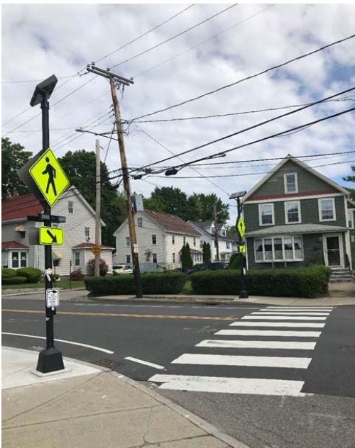
Left: Accessible crossing at River & Elm Streets - Rectangular Rapid Flashing Beacons (RRFB's)
