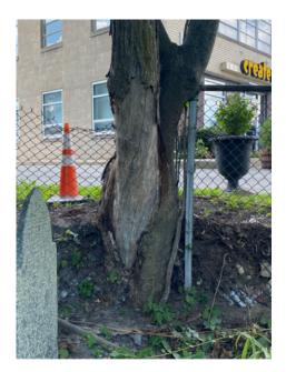
Before a new fence can be installed, the accumulated debris must be removed from the abutter's side of the fence in order to restore the original grade. If the original grade cannot be restored, a retaining wall will likely need to be built before installing the new fence.
