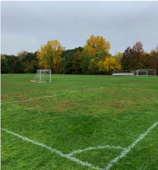
Left: Overall view looking Northwest: note brown patches which are low areas populated by weeds and voids.
