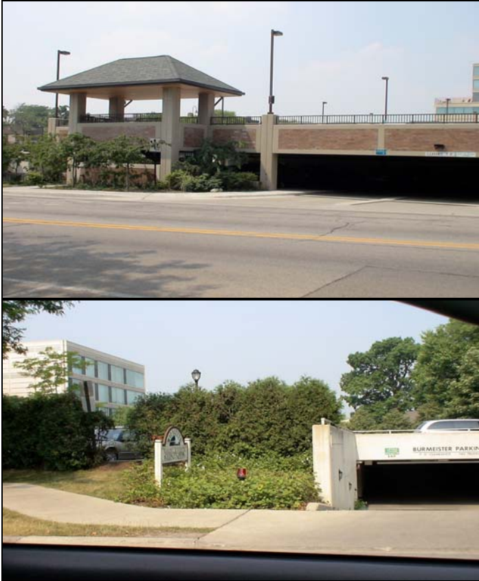
Some Examples of Well-designed Parking Structures
