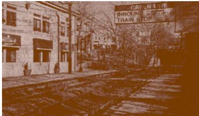
Newton Centre's "T" stop on the MBTA's "Riverside" Green line.
