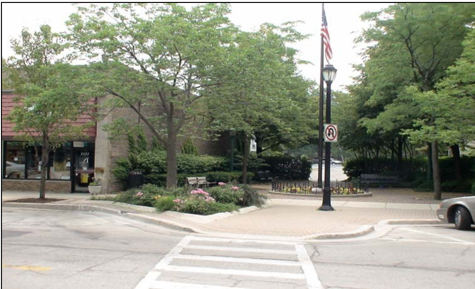
Curb bulb-out for traffic calming
