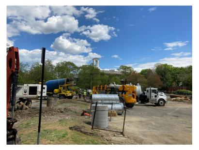
Ameresco began work this week literally laying the foundation for a "greener" Newton by installing foundation footings to support the solar carports being added to the Newton Free Library Parking lot on Homer Street. The solar panels will provide 40% of the library's electricity, and the new parking lot will include 21 more spaces including eight electric vehicle charging spots and will improve accessibility.
