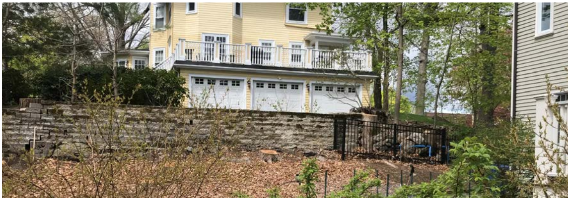
View of existing retaining wall along western property line.
