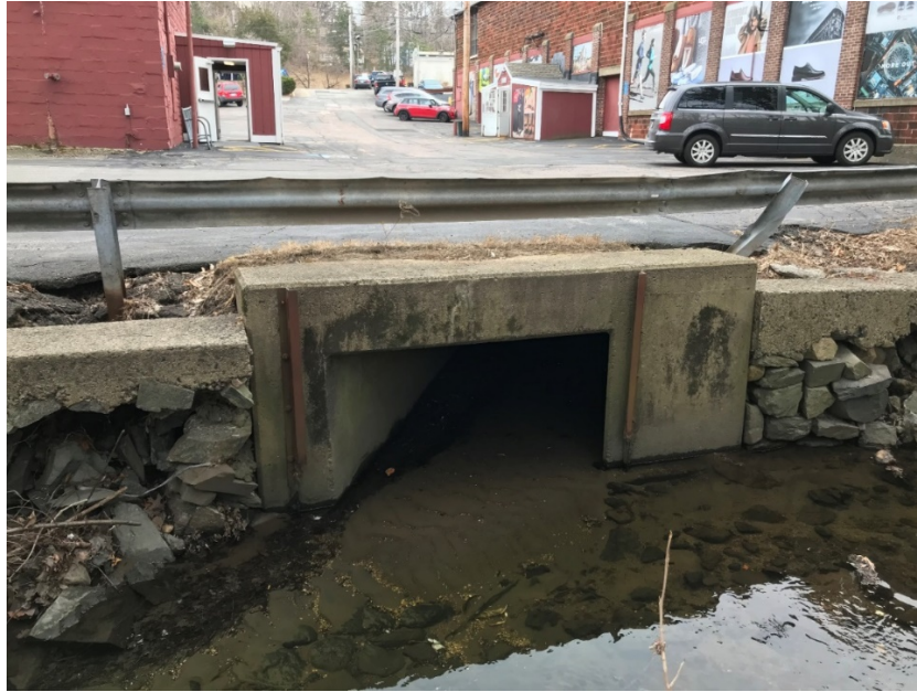
Existing Box culvert at Cheesecake Brook
