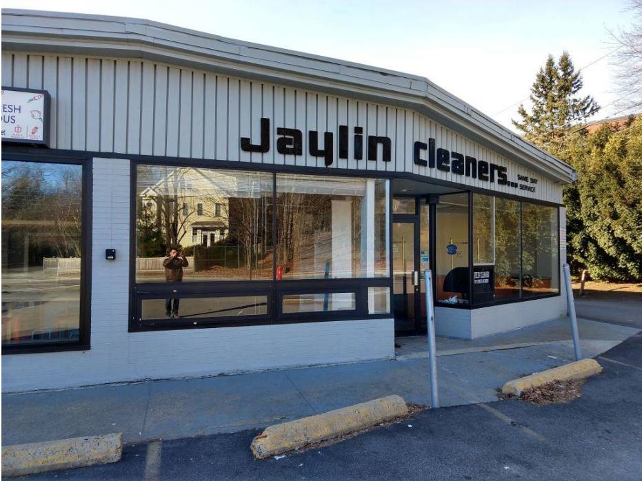
View of the proposed structure to be demolished from the north side [front of building]
