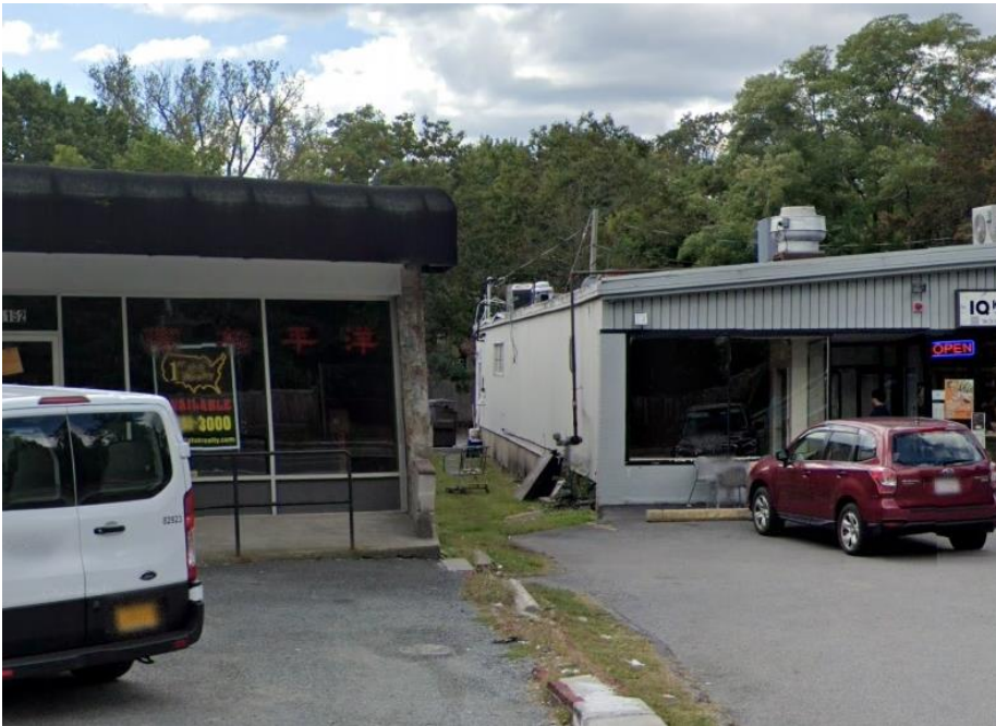
View of the proposed structure to be demolished from the north/east side [front and side of building]
