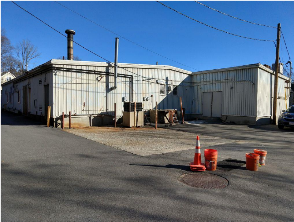
View of the proposed structure to be demolished from the south side [rear of building]
