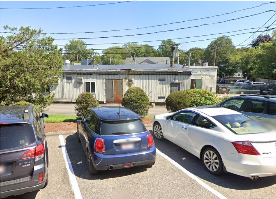
View of the proposed structure to be demolished from the west side [side of building]
