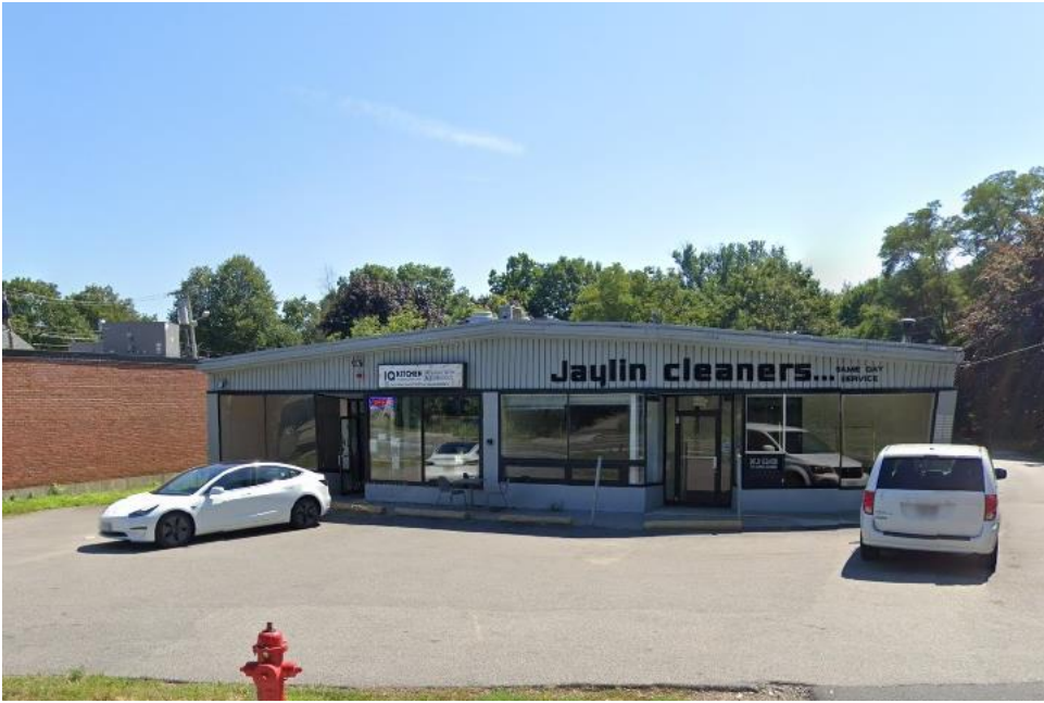
View of the proposed structure to be demolished from the north side [front of building/street view]
