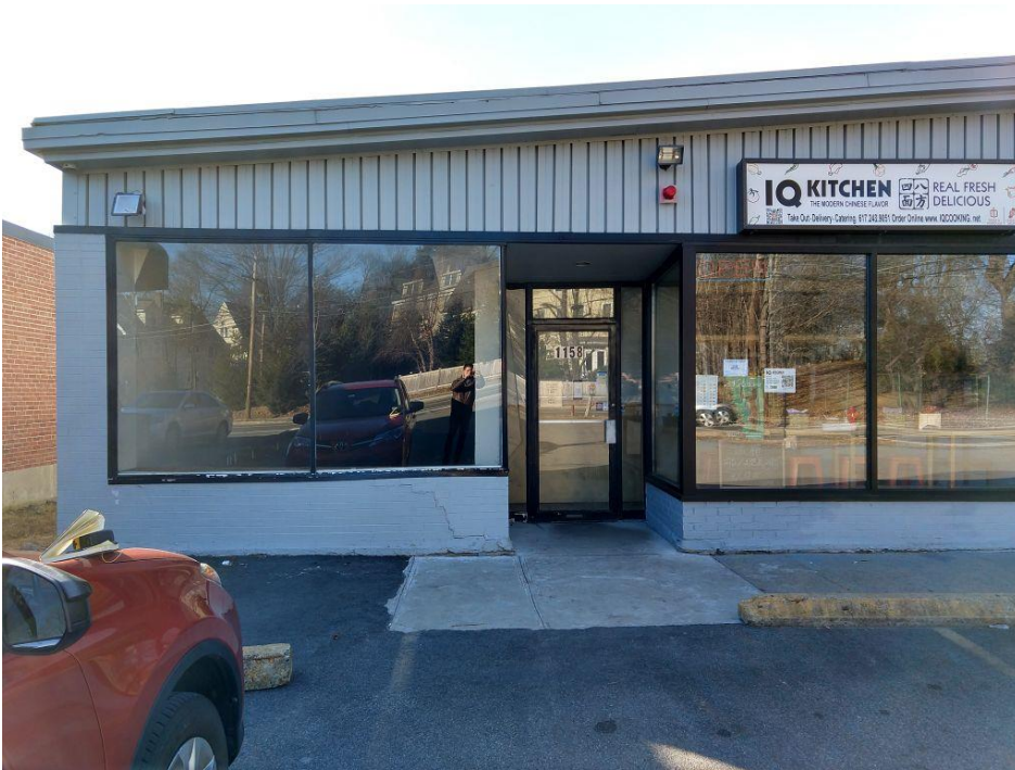
View of the proposed structure to be demolished from the north side [front of building]
