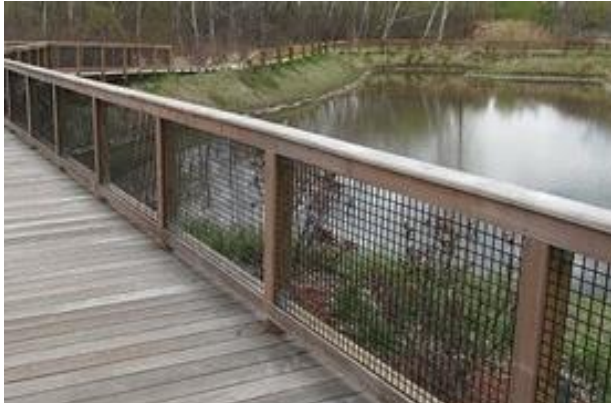
CANTILEVERED DECK SAFETY RAILING
