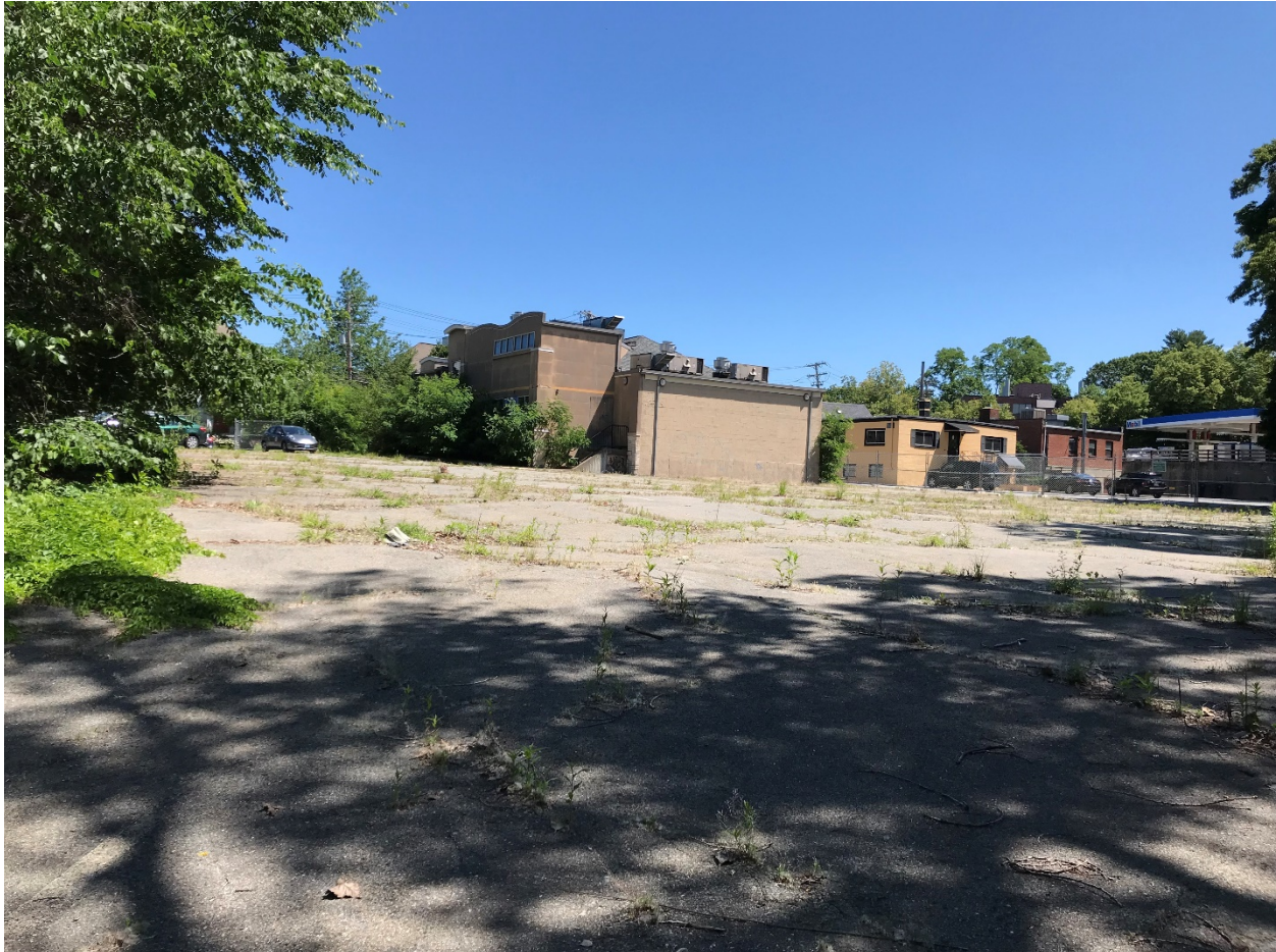
Looking North ~Existing parking lot & roof that sheet flows to the ILSF photo taken by J. Daghlian 6/17/21
