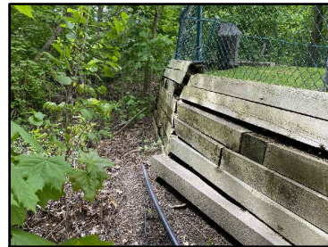
EXISTING RETAINING WALL ON NORTHEAST FACE
