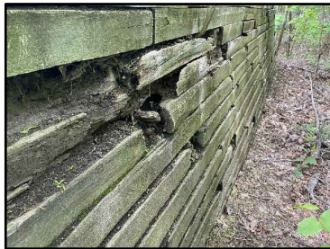
DETERIORATED WALL SECTION ALONG SOUTH FACE
