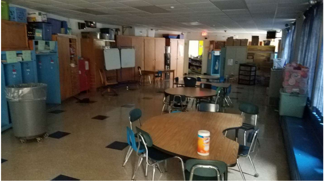
This is the lobby in the 1953 addition. As you can see, the classrooms being slightly undersized, has led to storage in the lobby.
