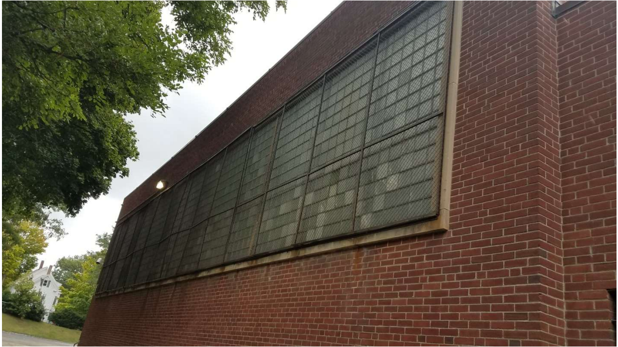
These are the original windows in the 1950 gym.
