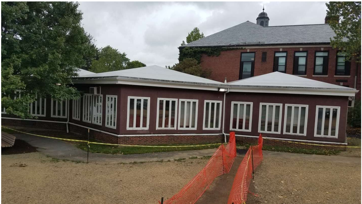
These windows were installed in 2000 in the 1950 addition.
