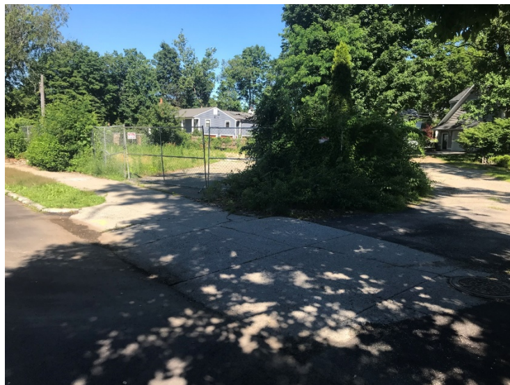
Existing common driveway apron
