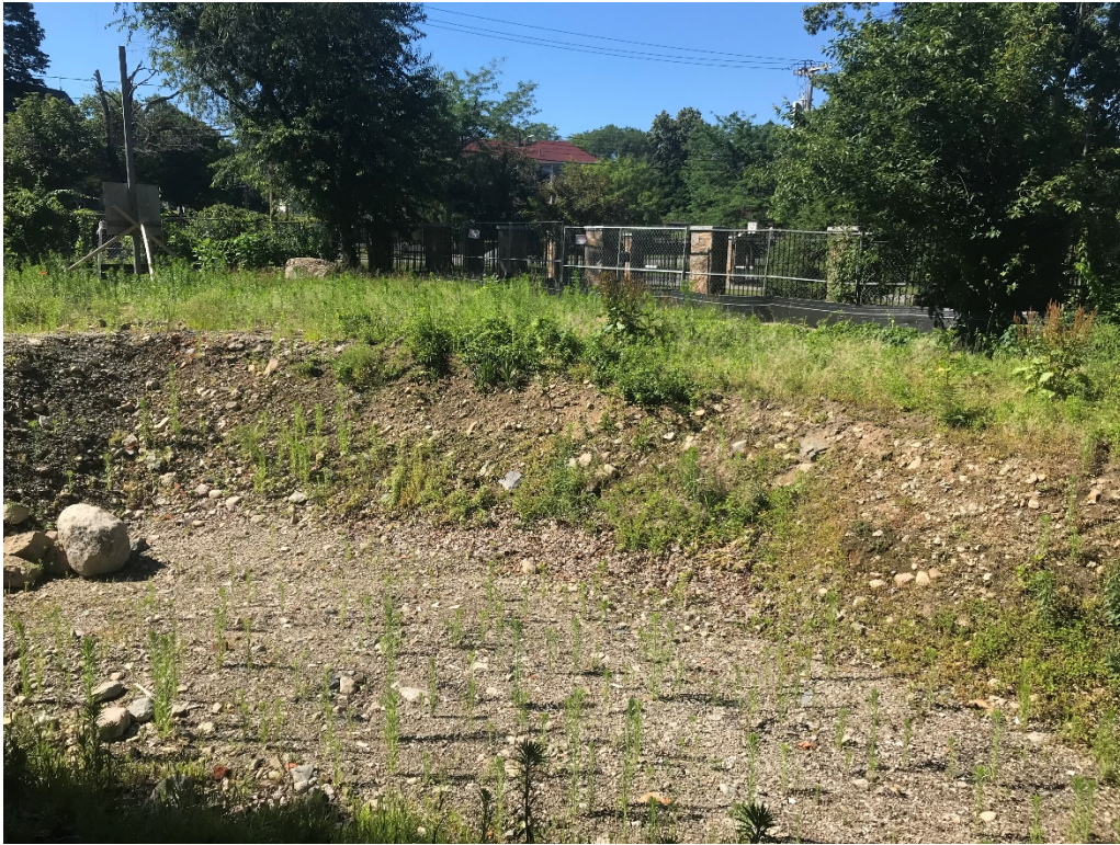
Existing dwelling razed photo taken: 6/24/2021.
