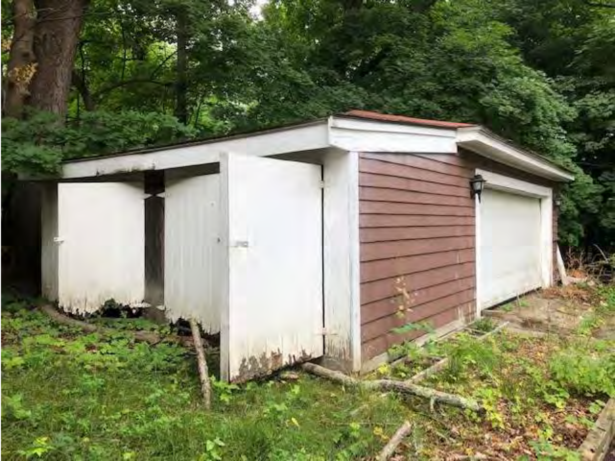
145 Warren Street, view looking northwest, detached garage addition
