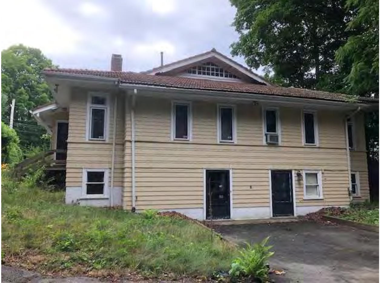
145 Warren Street, view looking south, rear facade
