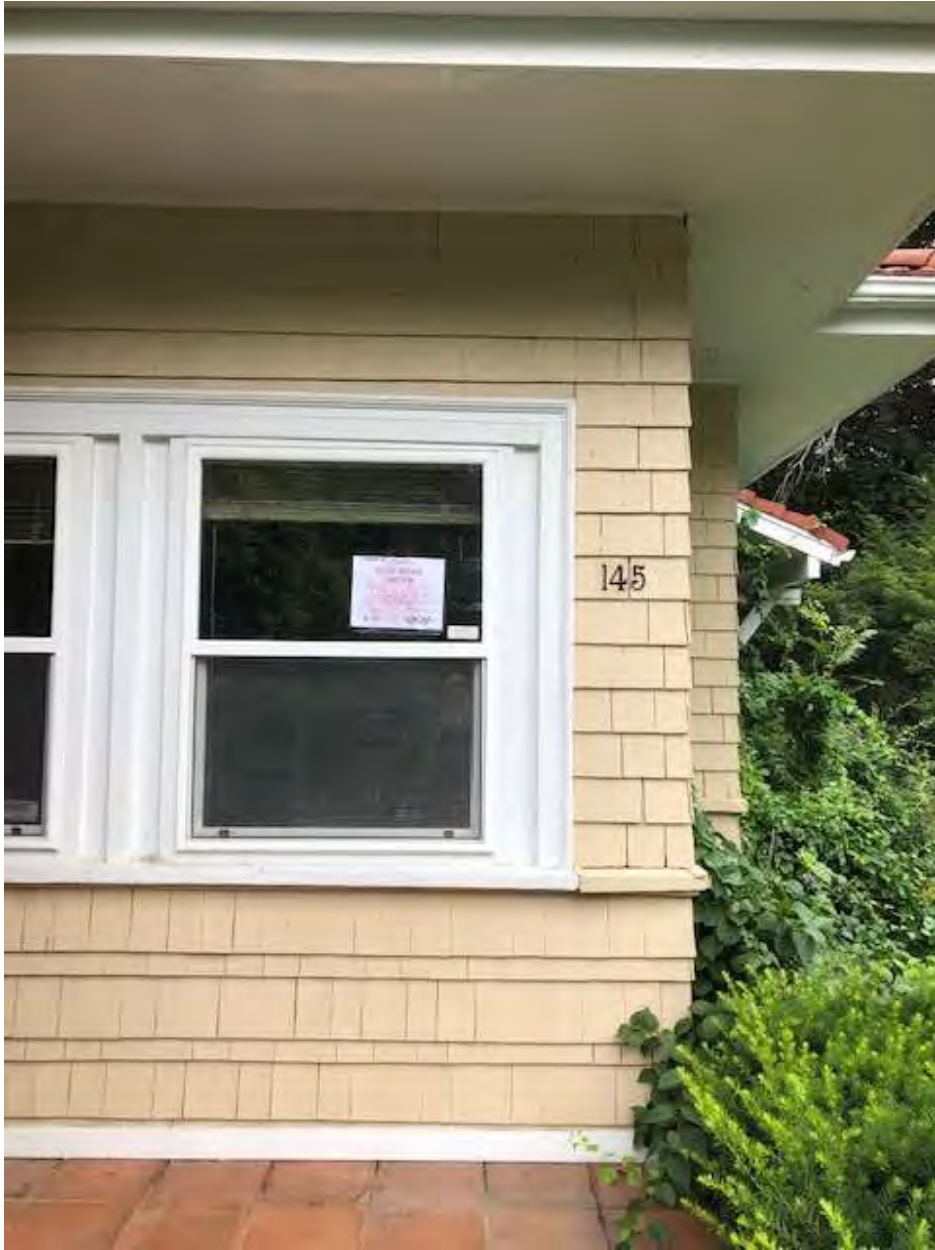
145 Warren Street, view looking north of front left corner
