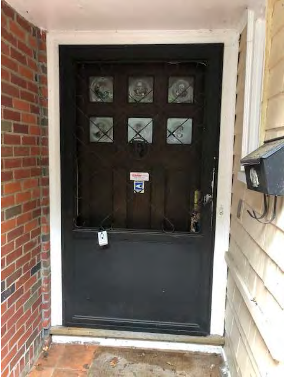
145 Warren Street, view looking north, front door
