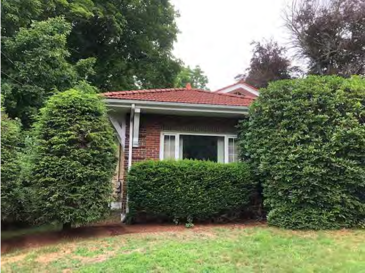
145 Warren Street, view looking north, front left façade, brick addition
