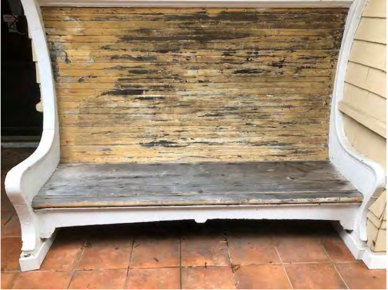
145 Warren Street, view looking west, front bench
