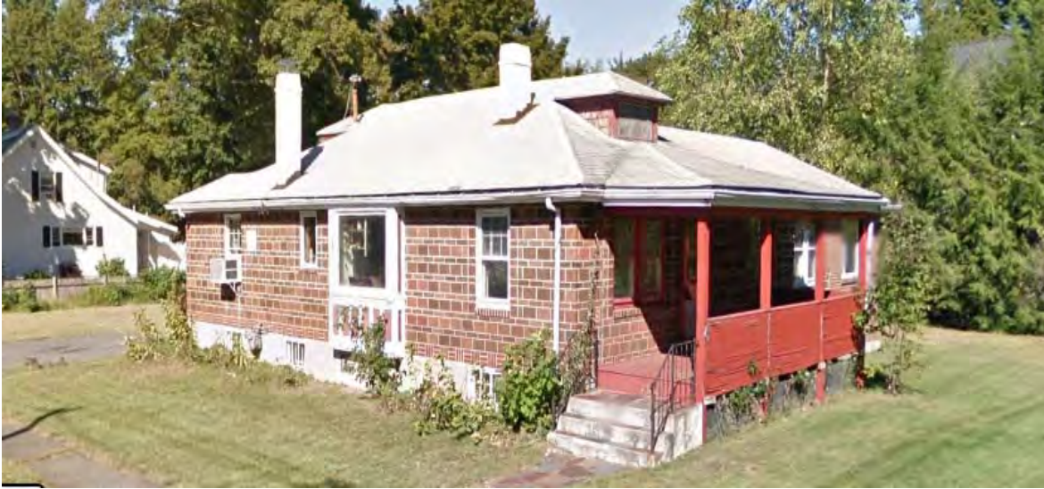
394 Weston Road, Hawley W. Morton (1921)
