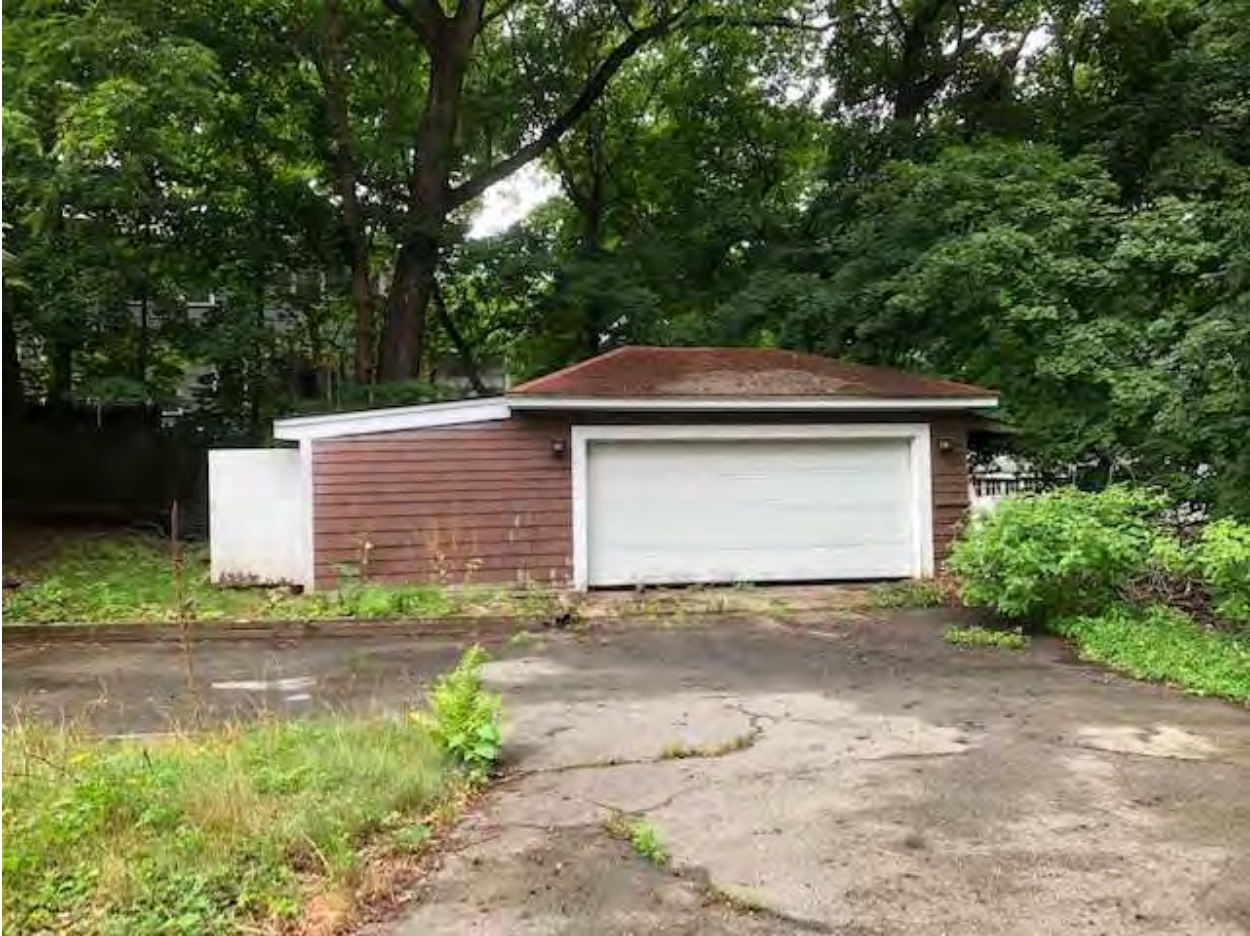
145 Warren Street, view looking west, detached garage
