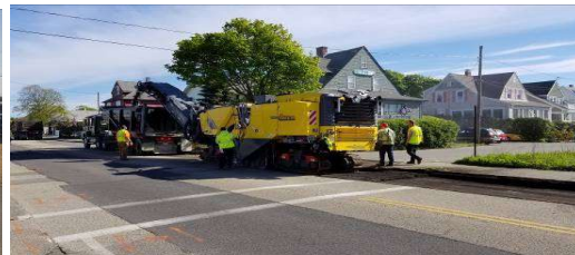
Mill and Overlay
