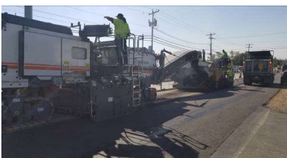
Cold In-Place Recycling
