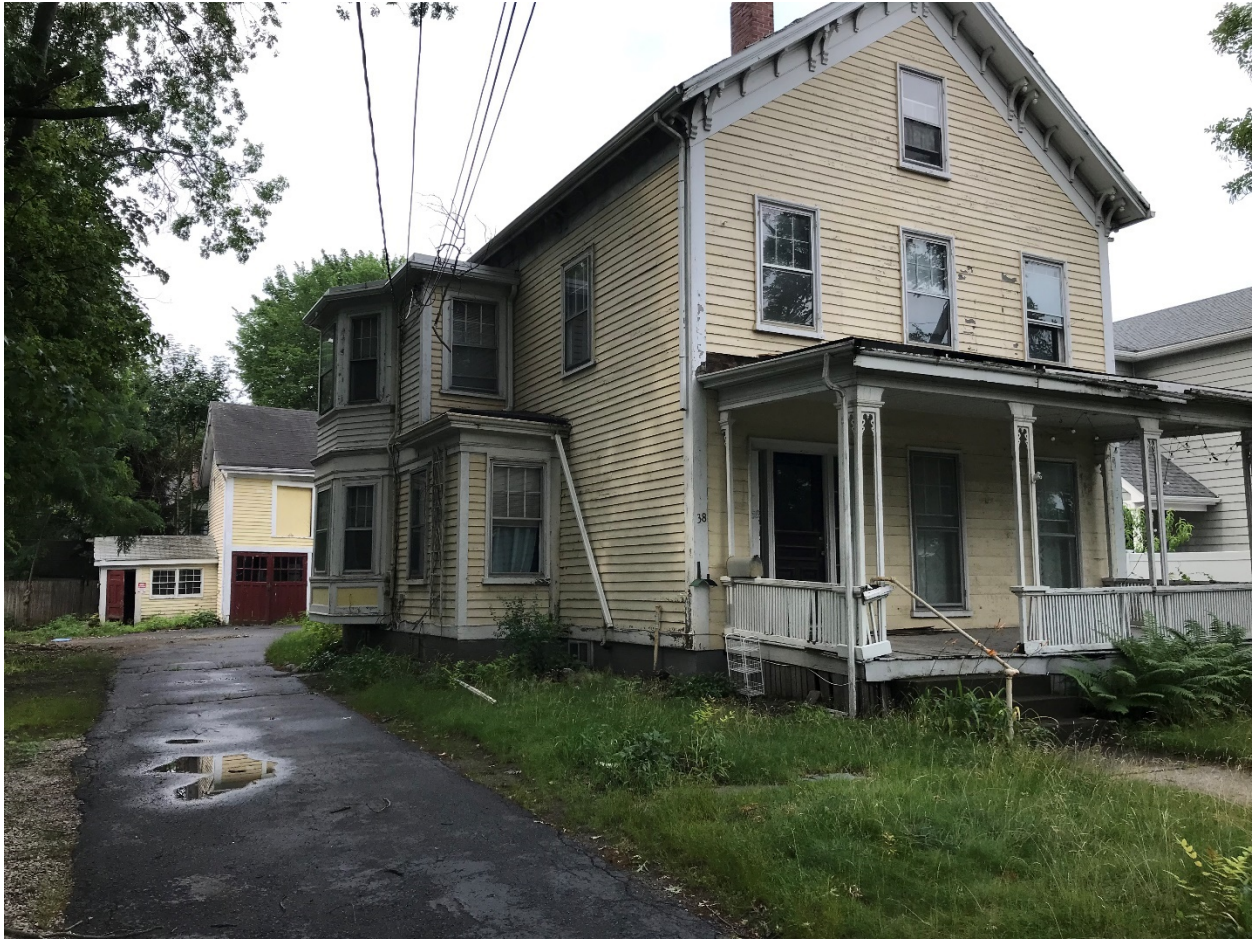
Detached garage to be razed.
