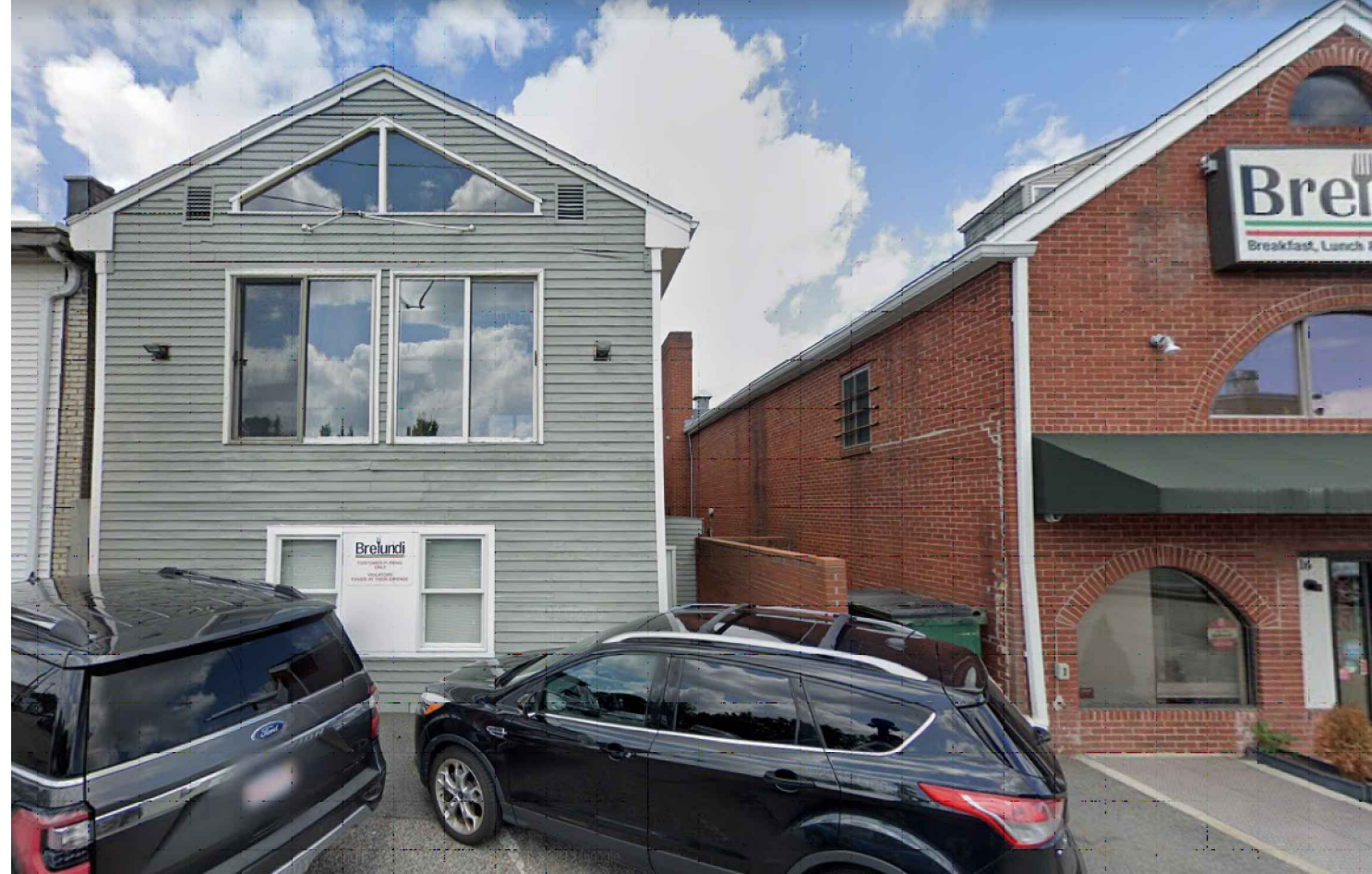
VIEW OF 20 FELTON STREET FROM RAILROAD PARKING LOT LOOKING NORTH
