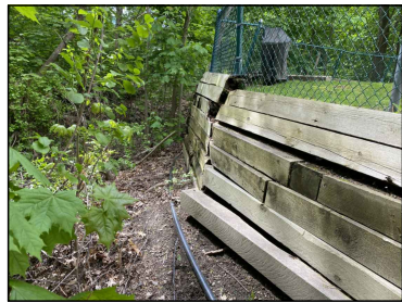
EXISTING RETAINING WALL ON NORTHEAST FACE 3
