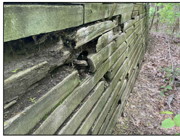
DETERIORATED WALL SECTION ALONG SOUTH FACE 3
