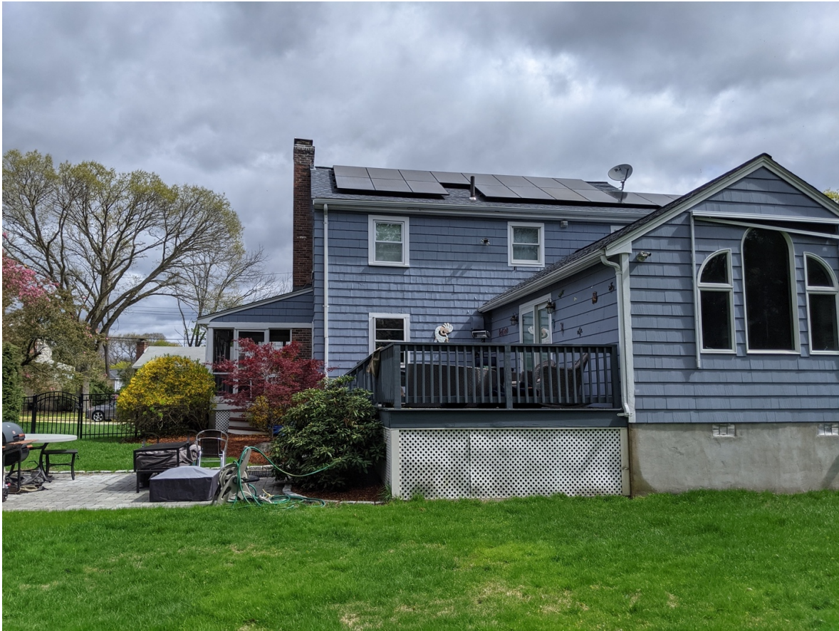
Figure 1. Location of the proposed addition, deck and patio to the left of the image, on the Northwest side of the house.
