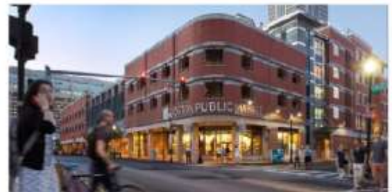
Ground floor commercial liner in parking structure
