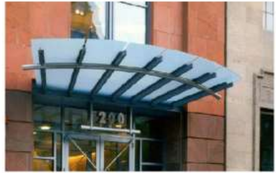
Added architectural detail at building entries
