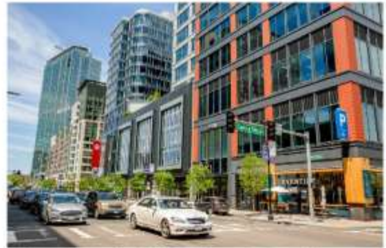
High quality and well-detailed use of materials
