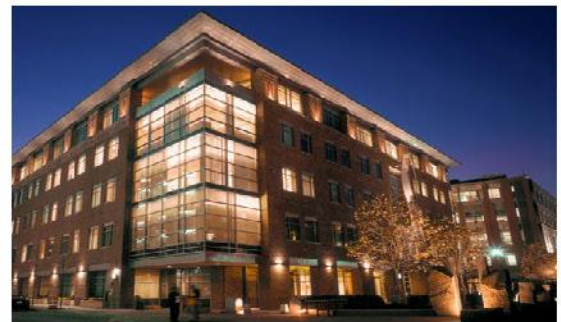
Highlighting architectural features of a building
