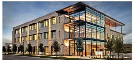
Highlighting architectural features of a building
