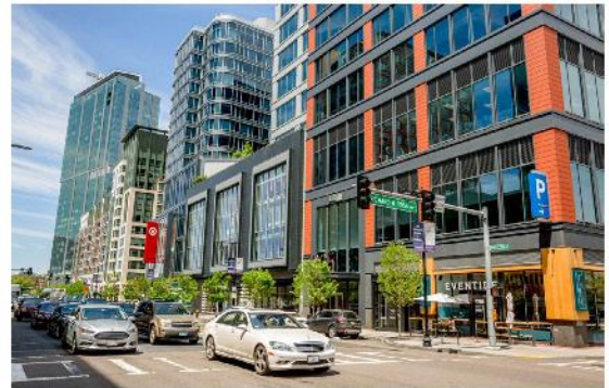
High quality and well-detailed use of materials
