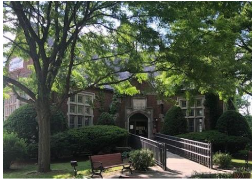
Photo of exterior entrance ramp at the Auburndale library
