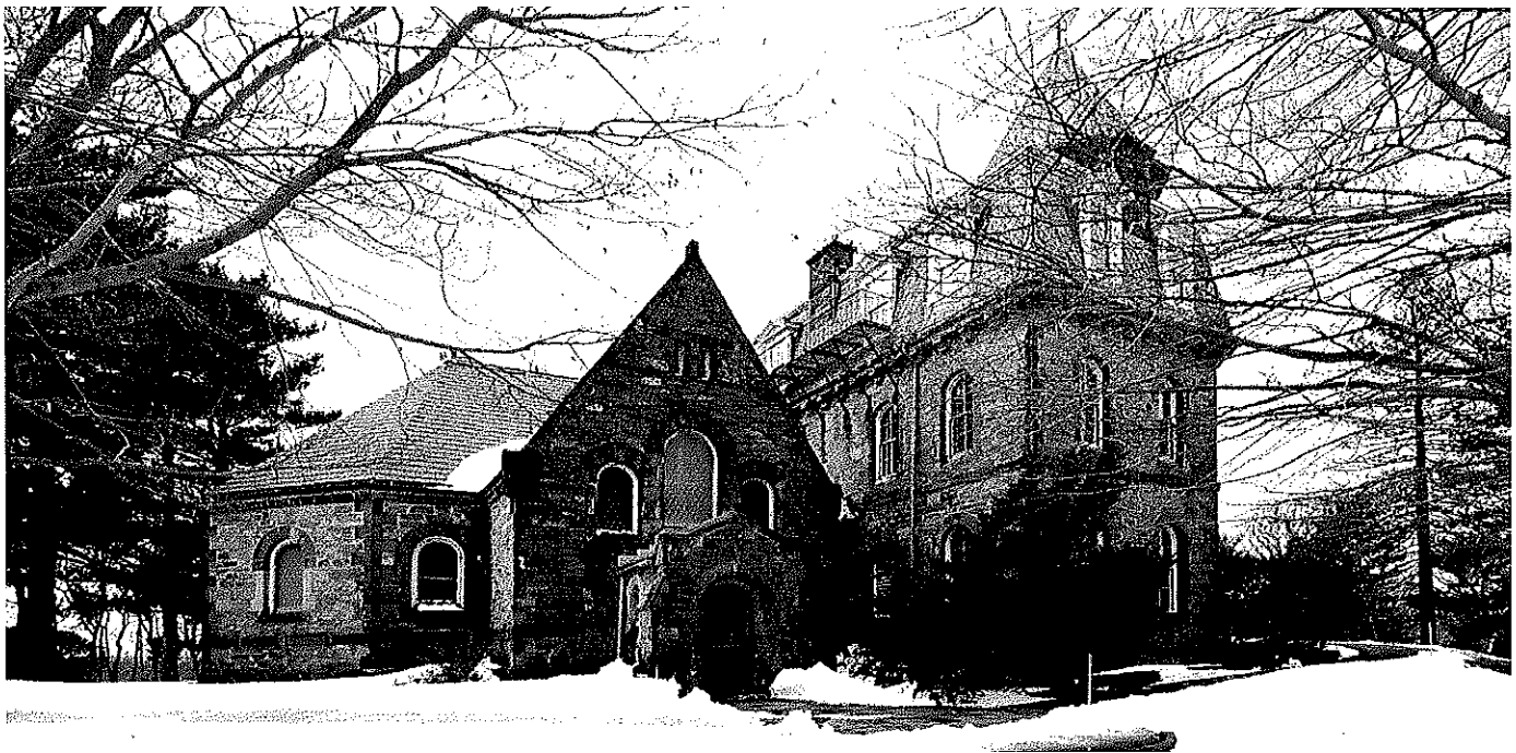
View of Chapel from southeast
