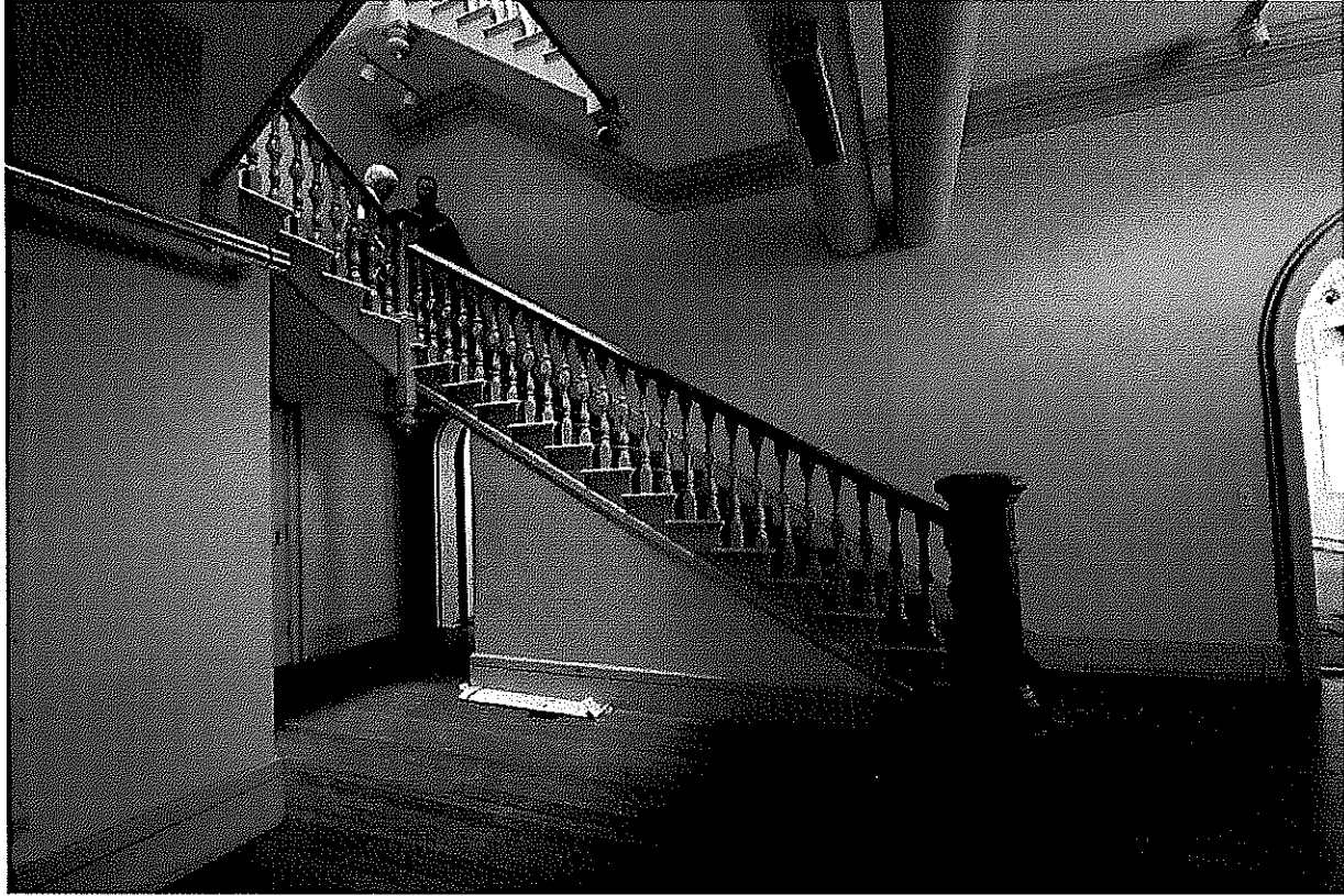
14] Photograph of Existing Interior Stair. Carpeting to be removed & existing nosing underside trim to be kept.
