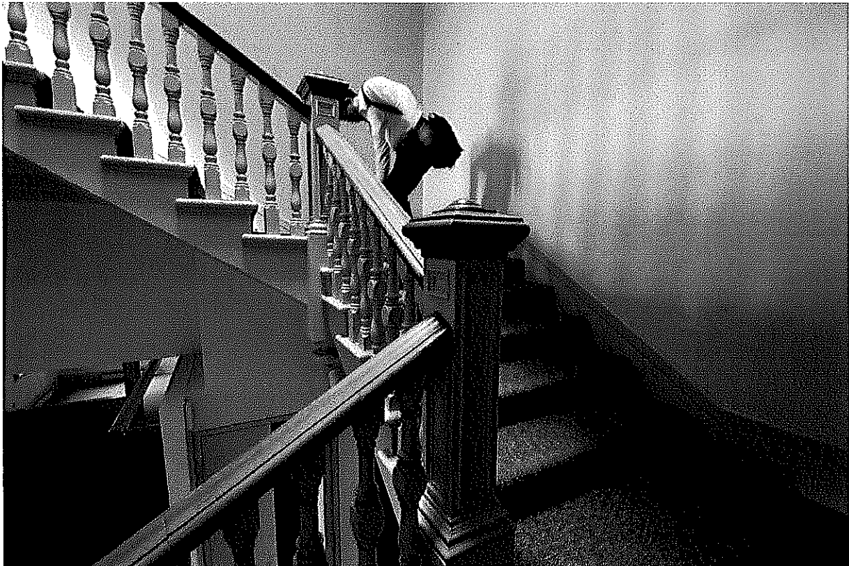
14] Photograph of Existing Interior Stair. Carpeting to be removed & existing nosing underside trim to be kept.
