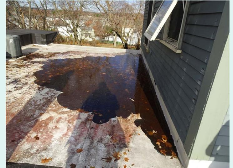
Existing roofs must be replaced. The new roof insulation will be increased to R-50, and the new roof will be a white TPO. The existing apartment air conditioning condensers must be removed and all 35 units replaced. These will be replaced with heating/cooling heat pumps to reduce green house gas emissions. Three gas fired Roof Top Units (RTU's) that cool the common areas will be replaced with higher efficiency equipment.
