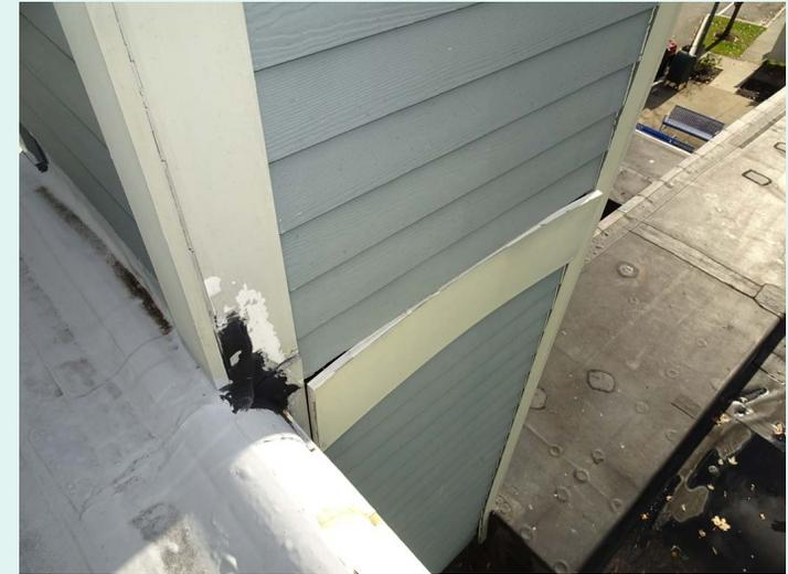
Sections of the siding and trim have extensive damage and must be replaced.
