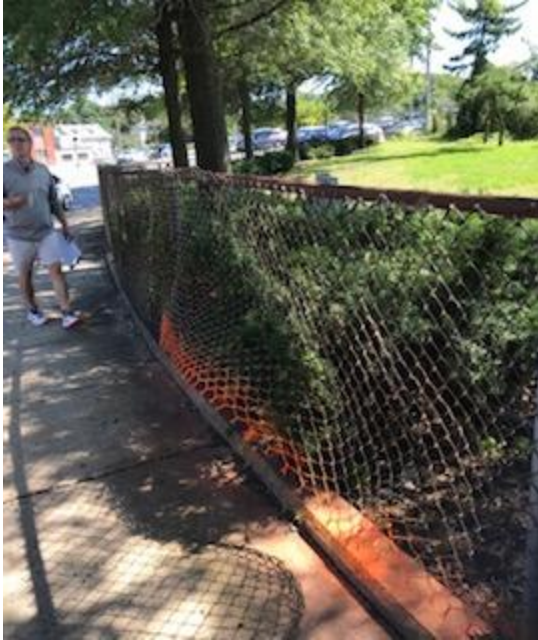
14. Unsafe, inaccessible sidewalks along the inner circle of the rotary.
