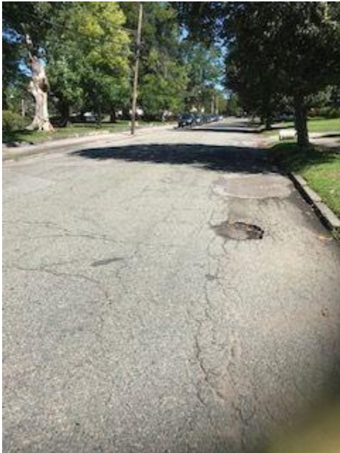
6. Repave surrounding streets.
