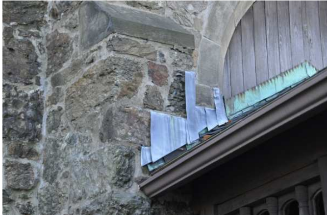
Photo 9: Flashing at Porte-cochere
