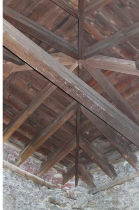
Photo 14: Wood ceiling structure in tower
