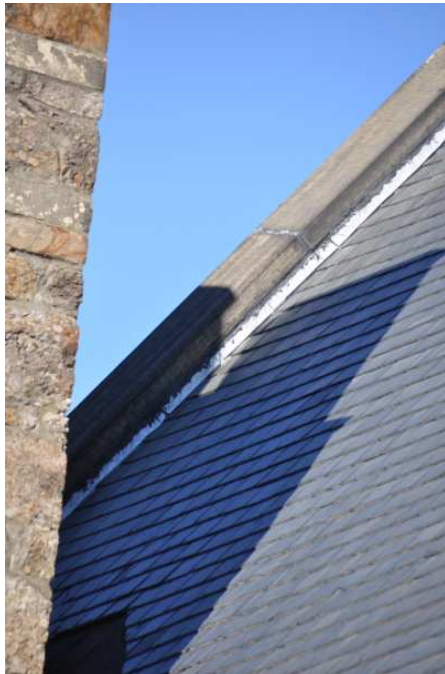
Photo 1: Flashing at Parapet
