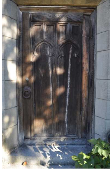
Photo 8: Entrance into Vestry
