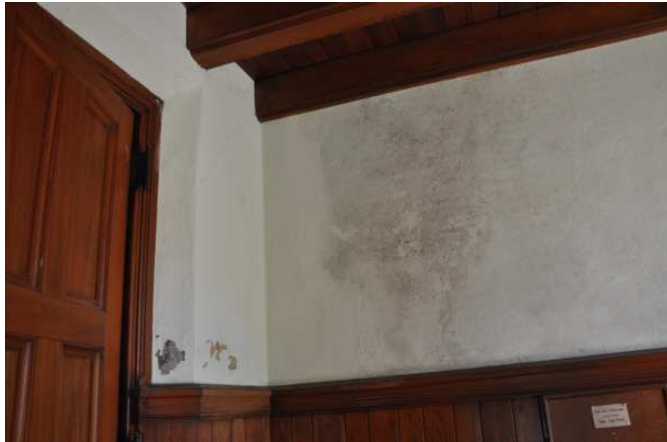
Photo 15: Wall in Vestibule
