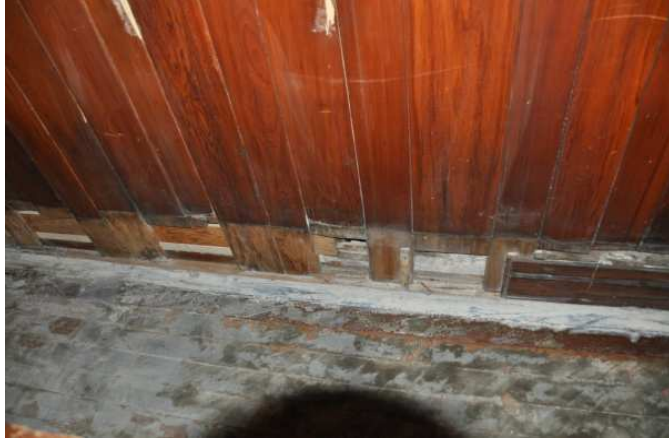
Photo 18: Wall and floor in Nave
