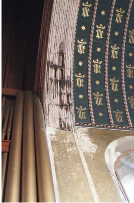
Photo 19: Arch in Chancel
