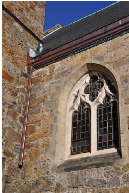
Photo 2: Downspout at Tower
