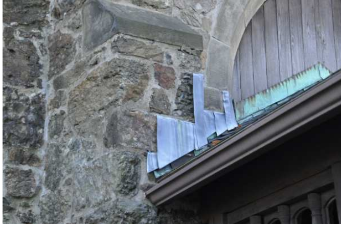
Photo 9: Flashing at Porte-cochere
