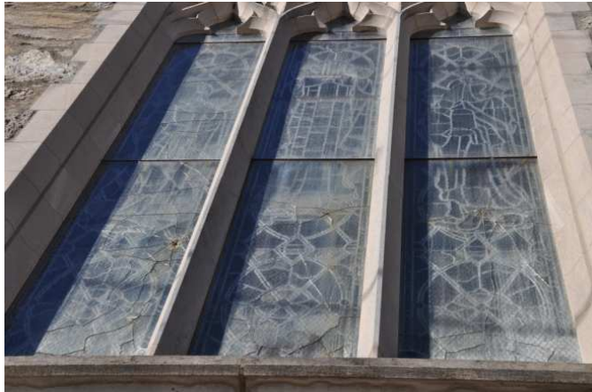
Photo 11: Protective Glazing at Altar Window
