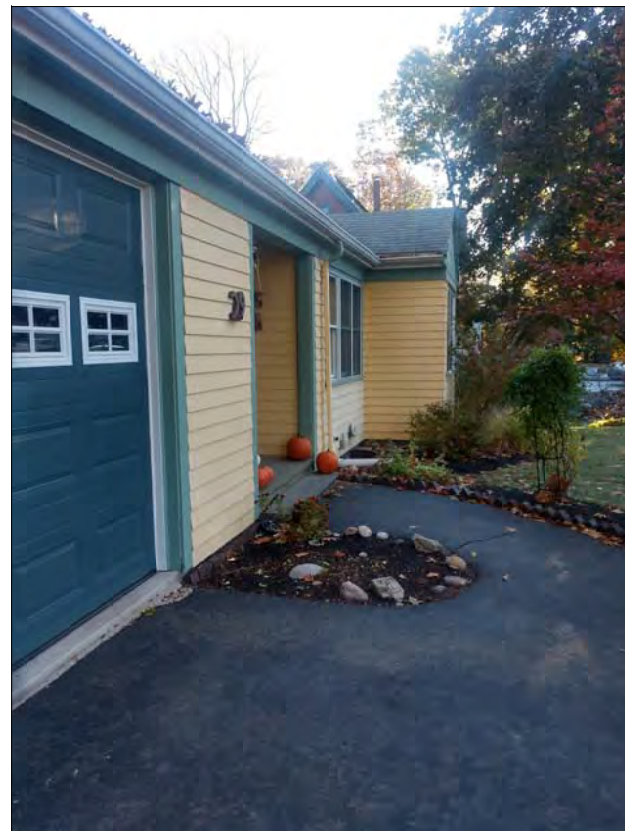
EXISTING FRONT ENTRY AREA
