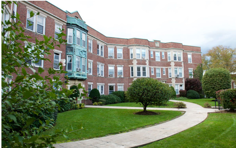
71-31 Herrick Road. This building is non-conforming under current zoning
