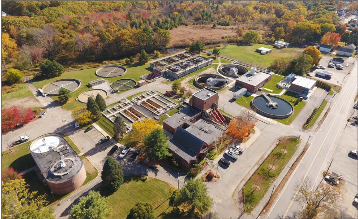
Clinton Wastewater Treatment Plant
