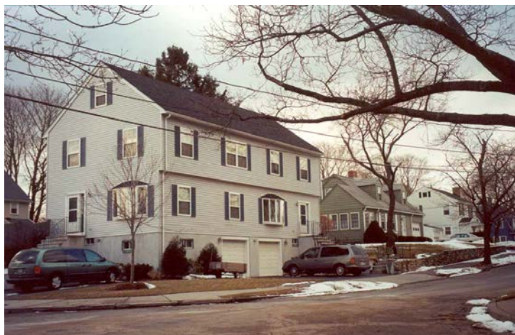
39 Fernwood Road – Feb. 2001
