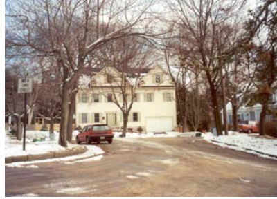
Replacement House at 11 Bunny Circle
