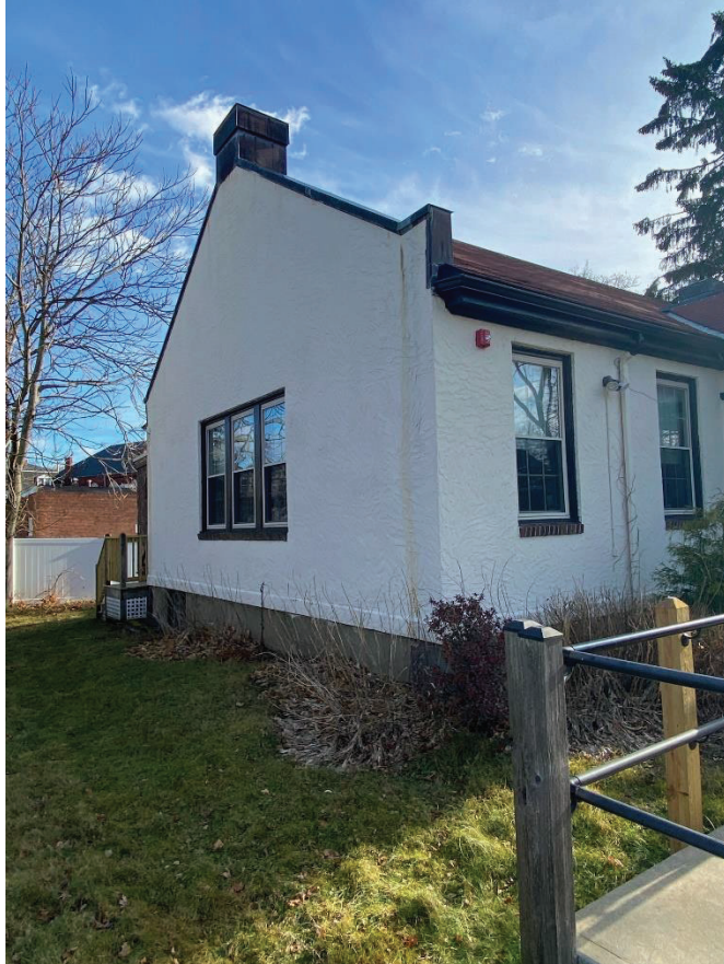
Photograph of the left side of the building
