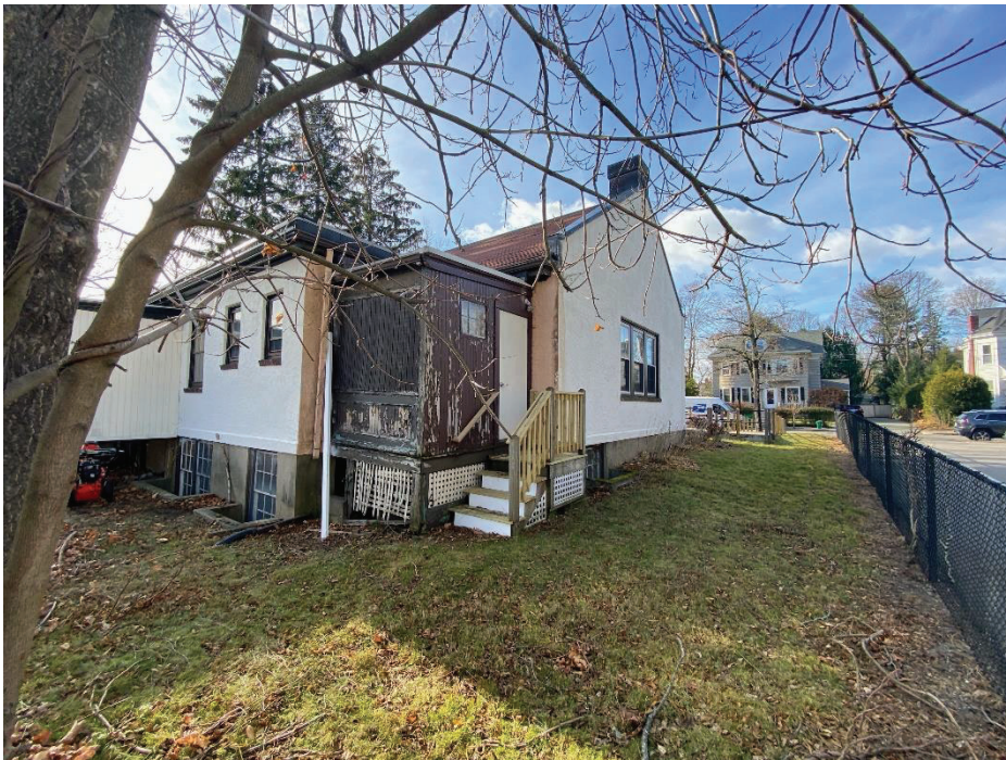
Photograph of a portion of the rear of the building
