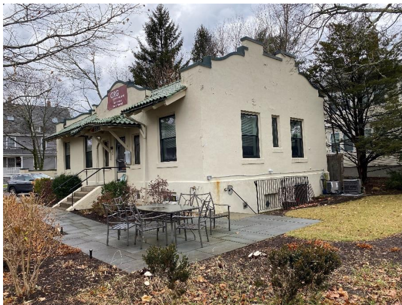
555 Commonwealth Avenue Newton, MA designed by Edward Stratton
