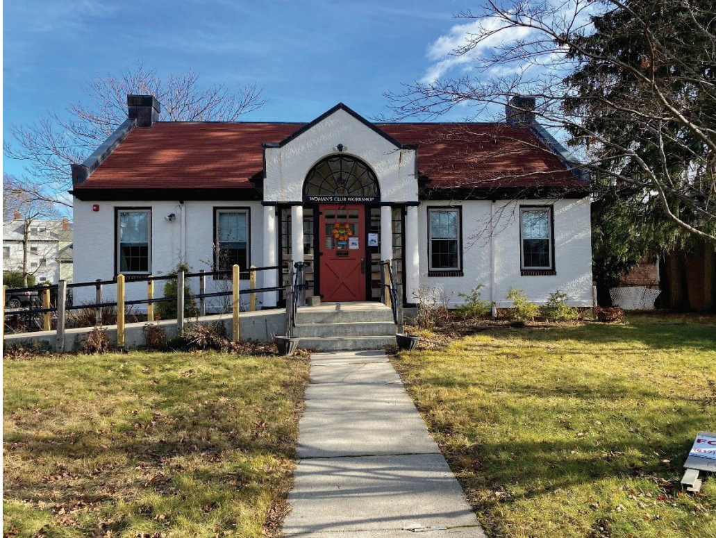
Photograph of the front of the building
