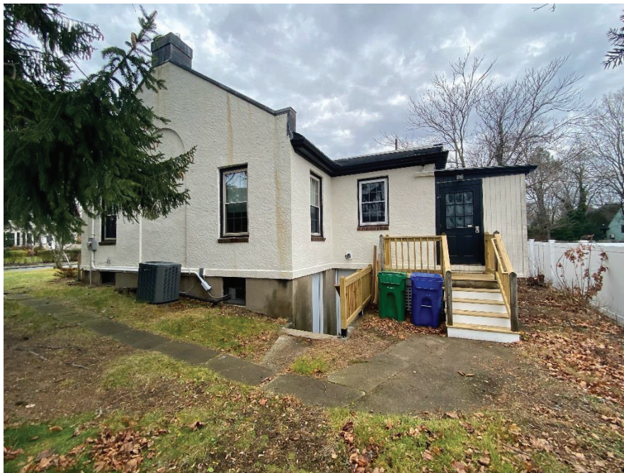
Photograph of the right side of the building
