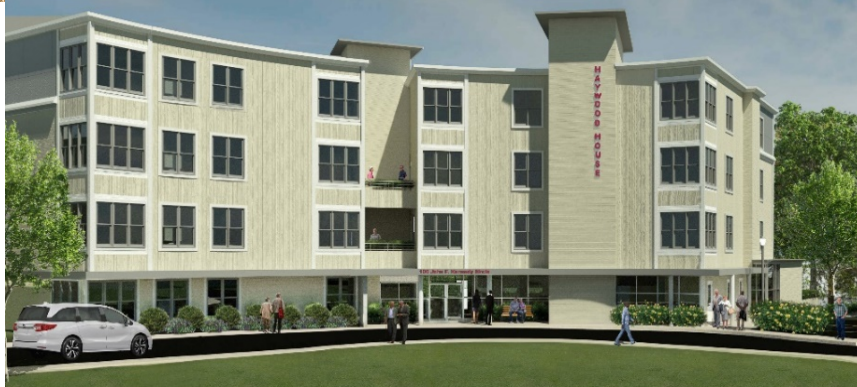
Haywood House Senior Affordable Housing Development
